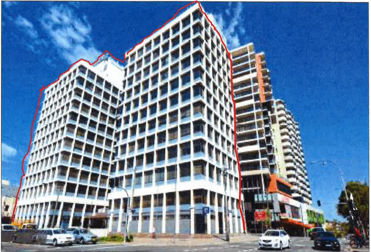
Figure 2: Site viewed from the north on corner of Gibbons Street and Lawson Square (Source: https://www.raywhitecommercial.com/ )
