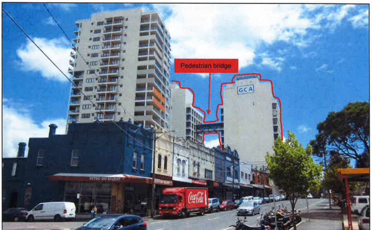
Figure 3: Site viewed from the south on Regent Street showing rear façade of towers (Applicant's EA for SSD 5249)
