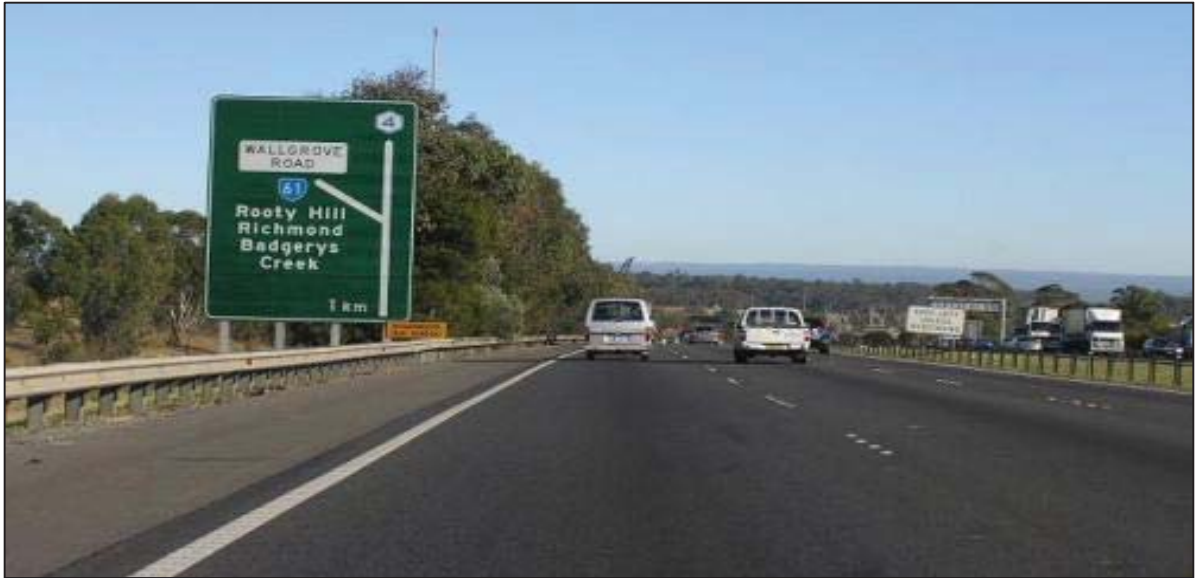
M4 Westerns Motorway viewed westward approaching the Old Wallgrove Road ramps
