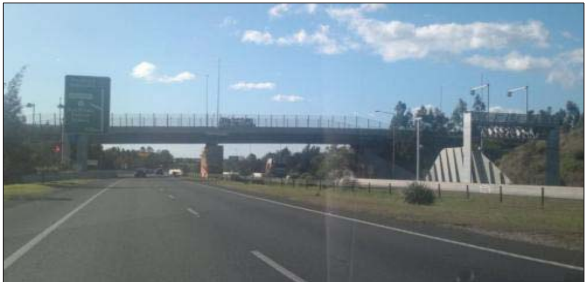
Westlink M7 Motorway viewed northward approaching the Old Wallgrove Road (southbound) ramps
