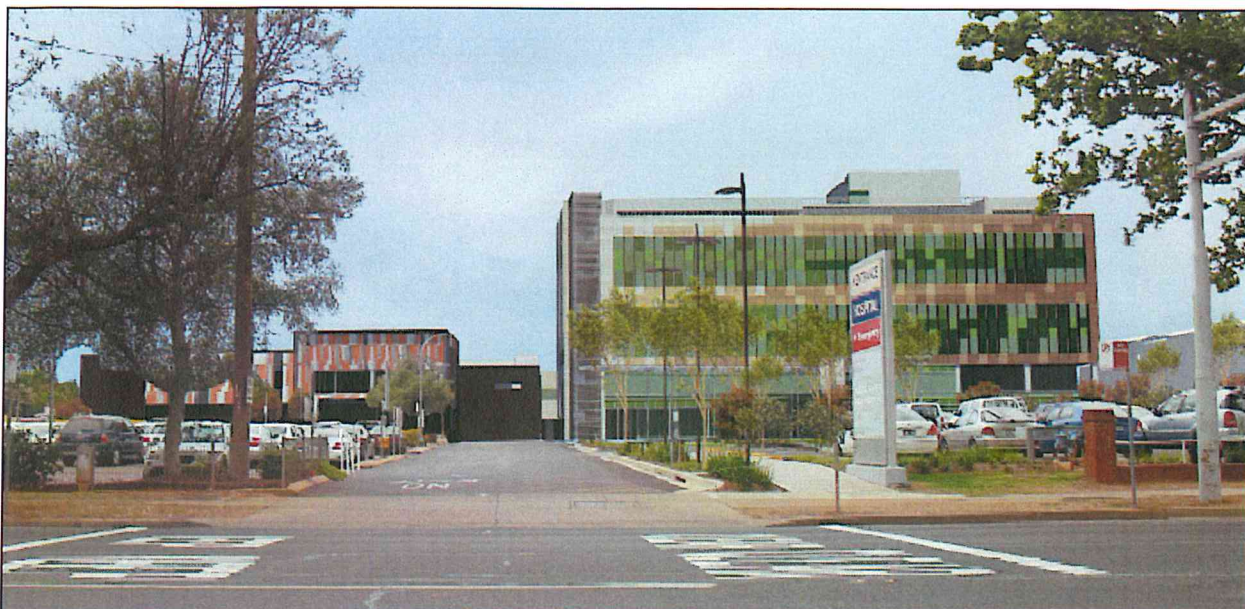
Figure 5: View from Edward Street – approved
