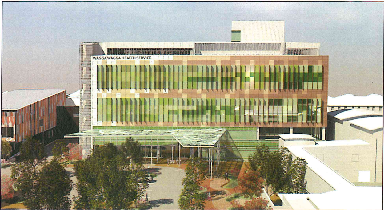
Figure 3: Aerial view from north – approved
