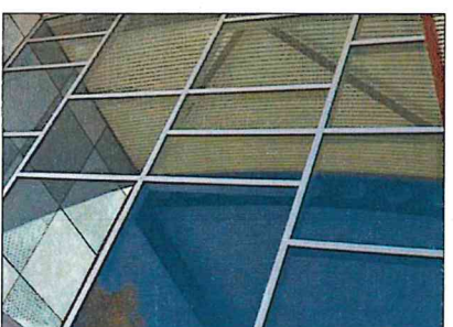
[GL1] GLAZING, WITH ALUMINIUM FRAMING PANELS: TRANSPARENT
