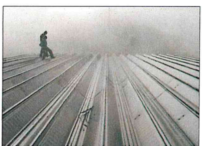
[RC] STRUCTURAL ROOF SHEETING, COLOUR: SILVER.
