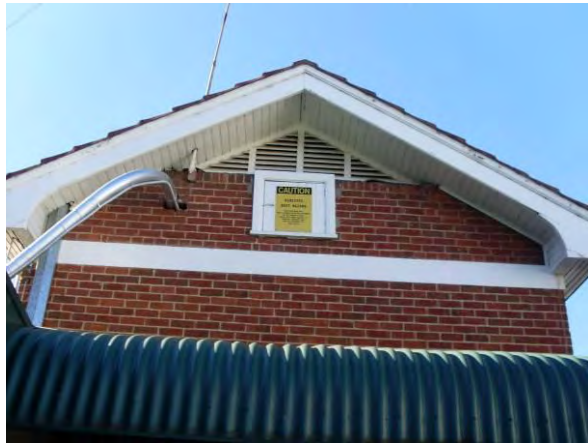
PICTURE 8 – THE SOUTHERN ELEVATION GABLE END.
