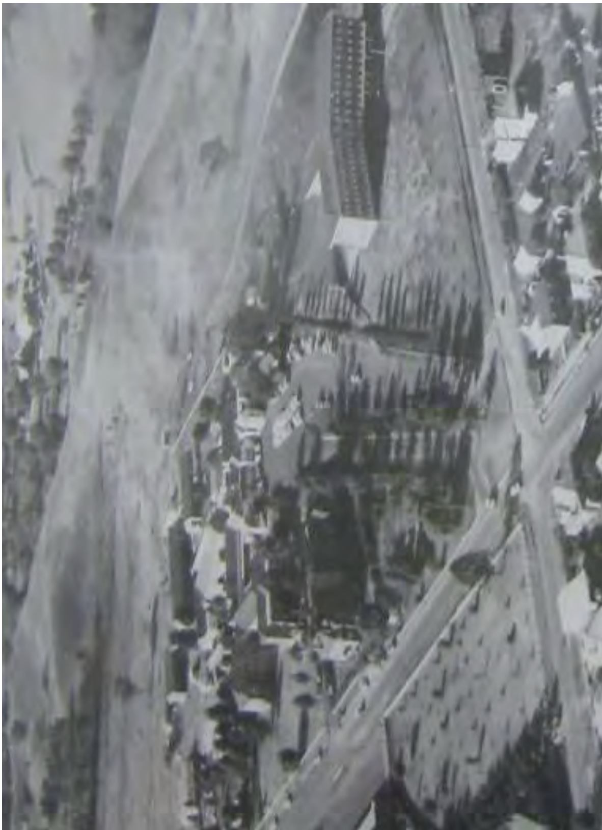
PICTURE 37 – 1965 AERIAL PRESENTED BY G.A SOLOMONS ESQ. ON THE OPENING OF THE NEWLY BUILT JOHNSTON HOUSE (SHOWN AT RIGHT). THE VIEW ALSO SHOWS SOME ADDITIONAL DEVELOPMENT IN THE NORTHEAST AND NORTHWEST QUADRANTS.
