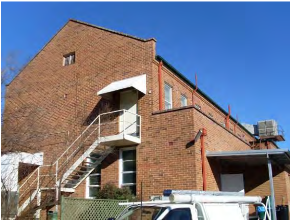
PICTURE 15 – NORTH ELEVATION
