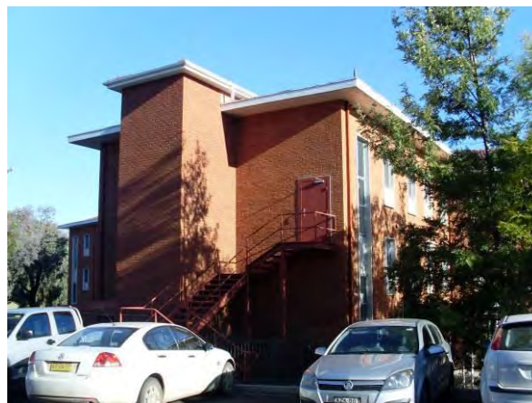
PICTURE 20 – THE NORTHERN WING (REAR).
