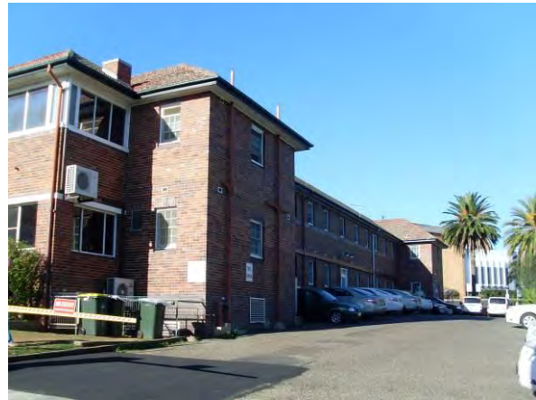
PICTURE 12 – SOUTHERN ELEVATION OF DEAN HOUSE,
