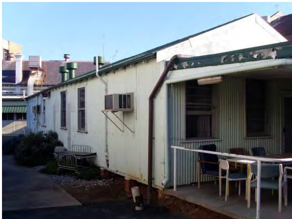
PICTURE 29 – VIEW OF THE NORTHERN AND EASTERN ELEVATIONS
