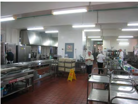
Picture 17 – Ground floor industrial kitchen servicing the patients
