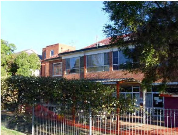
PICTURE 23 – NORTHERN ELEVATION OF THE CHILDREN'S WARD
