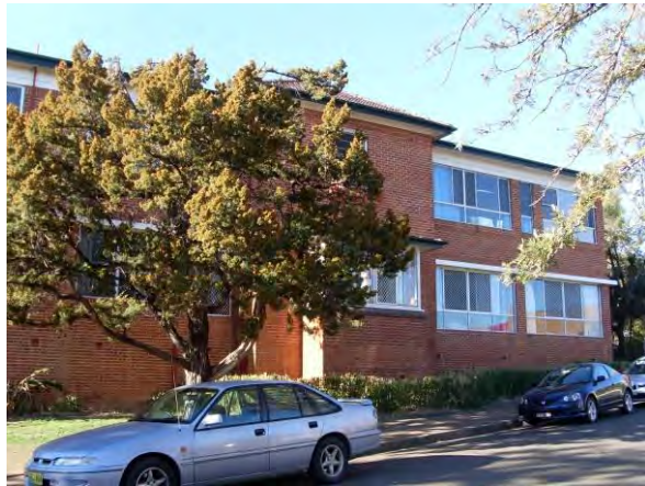
PICTURE 24 – PRINCIPAL SOUTHERN ELEVATION OVERLOOKING THE EXIT ROAD TO DEAN STREET. FAÇADE FEATURES INFILLED LOGGIAS.
