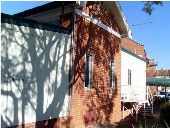
PICTURE 7 – WESTERN ELEVATION OF THE RENAL WARD WITH LEAN TO ADDITIONS FLANKING THE ORIGINAL BUILDING.
