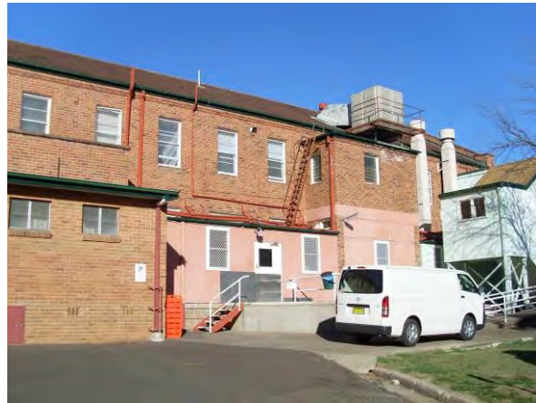
PICTURE 16 – VIEW OF THE WESTERN ELEVATION SHOWING ACCRETIONS.
