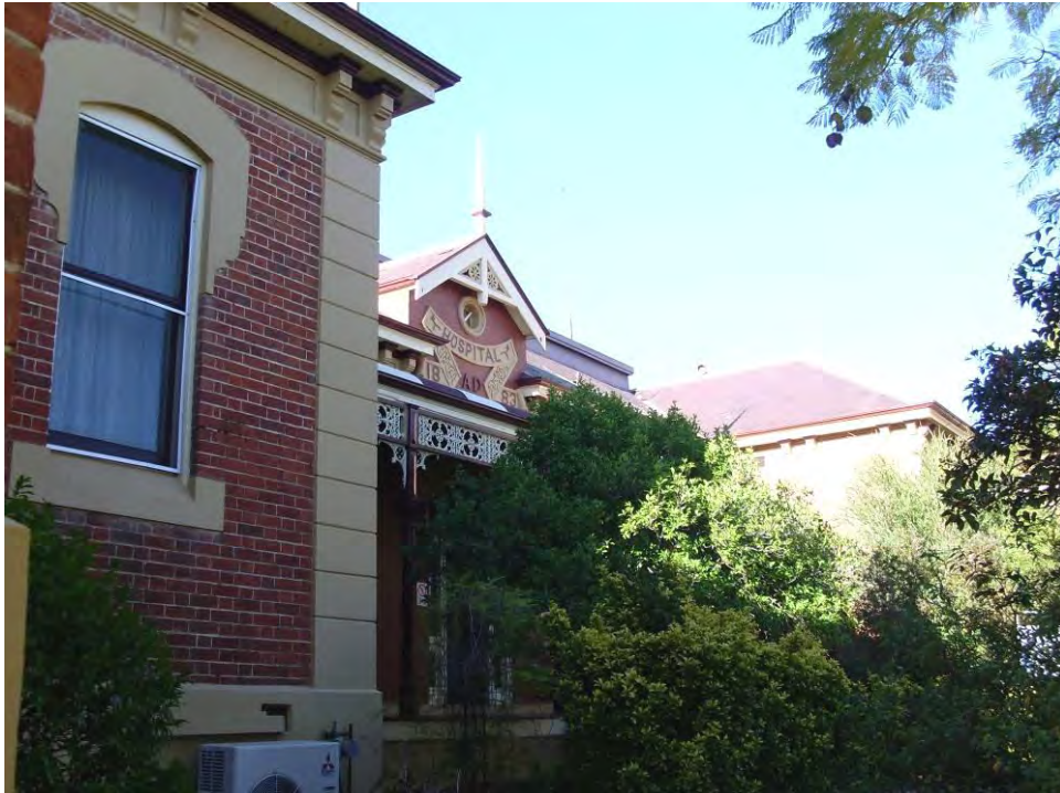
PICTURE 1 – PART VIEW OF THE ORIGINAL 1883 HOSPITAL
