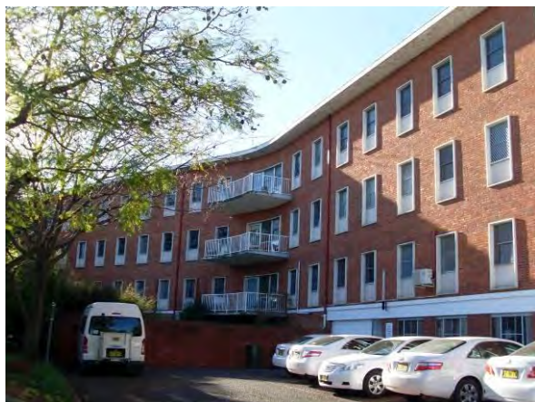
PICTURE 19 – THE SOUTHERN JOHNSTON STREET ELEVATION
