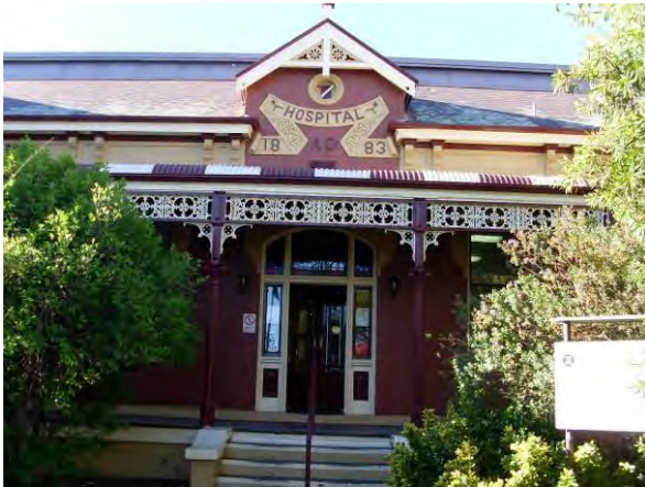
PICTURE 3 – THE PRINCIPAL ENTRY
