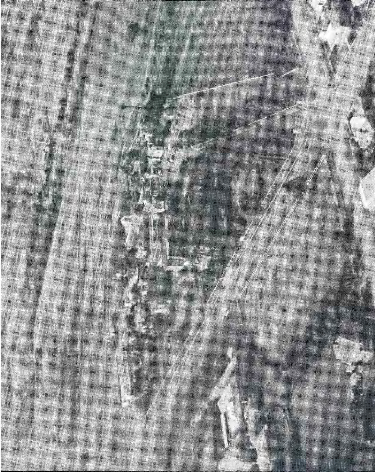
PICTURE 36 – 1957 AERIAL VIEW
