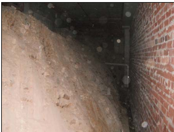
Figure 8: Existing cutting under Brudelin Wing at 0.6H:1V
