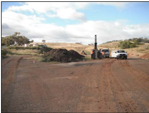
Figure 2: Drilling rig at Bore 109 with stockpiles on hospital boundary
