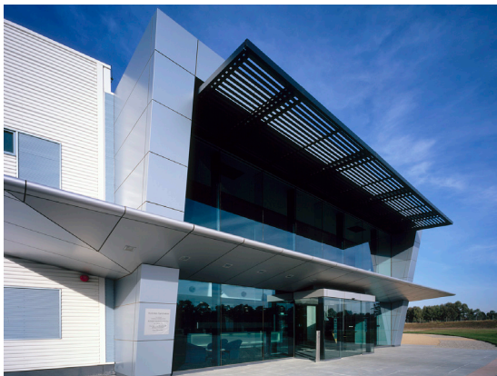
Figure 17: Bulky-goods-Specialised retail premises - Shade structures and awnings provide amenity and increase energy efficiency. Two to three materials are used simply and effectively to articulate the entry to the development.
