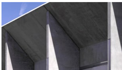
Figure 38-37: Exposed concrete is a durable material that can be used in a number of ways to articulate a building form.
