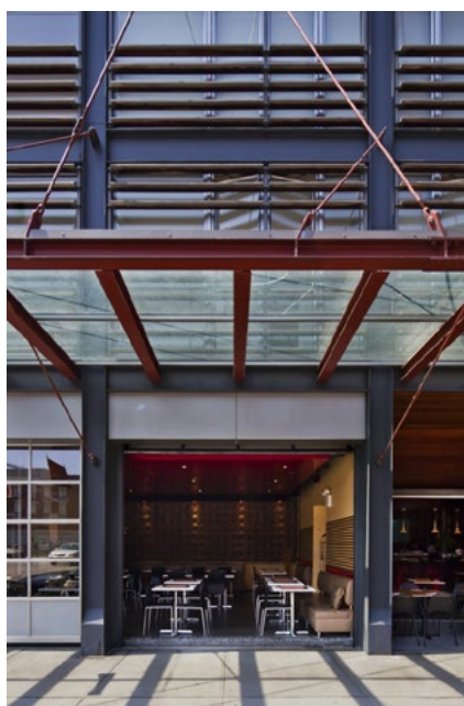
Figure 37-36: Exposed structural elements break down the bulk of a horizontal building form.
