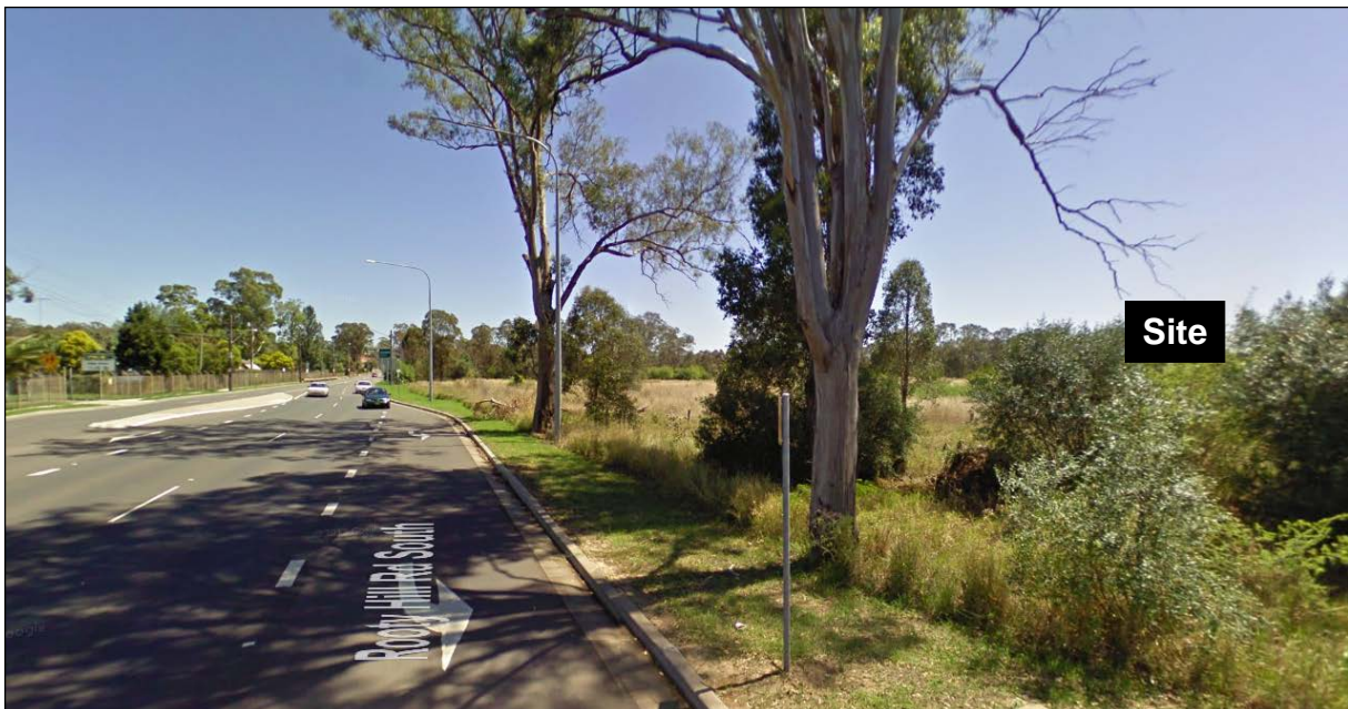
Figure 4: View looking north along Rooty Hill Road South
