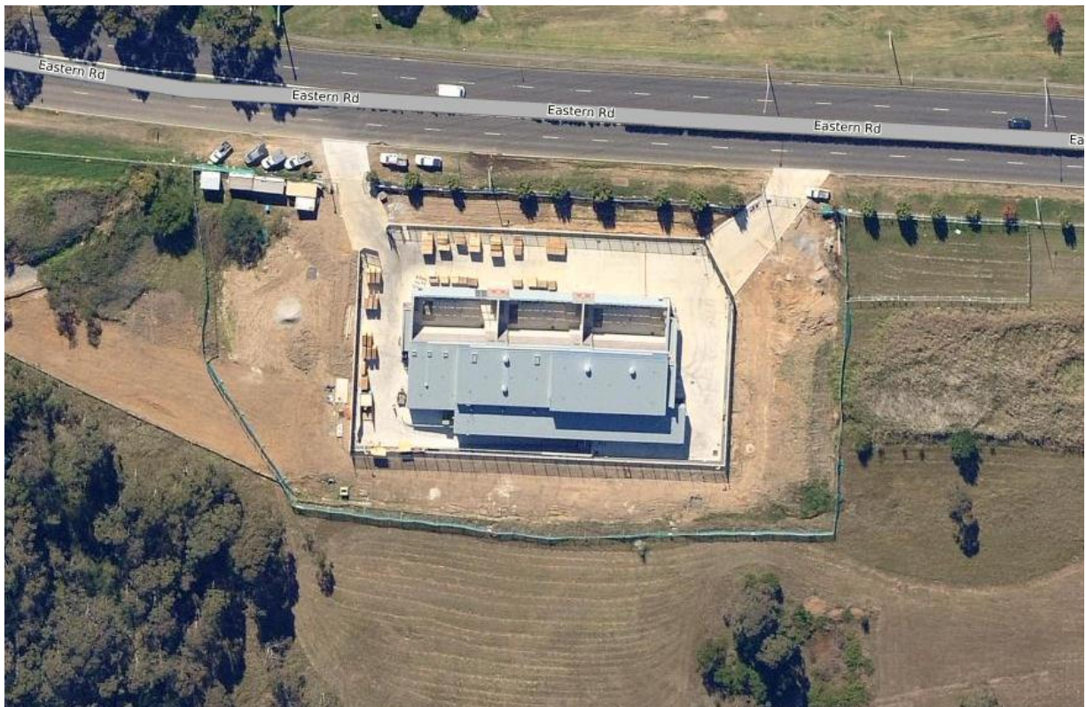
Figure 2 Zone Substation at 9 May 2012 (Source Nearmap)
