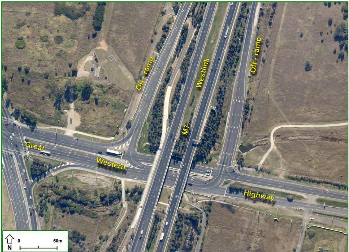
Figure 6: Intersection of the Great Western Highway with the Westlink M7 On/Off Ramps
