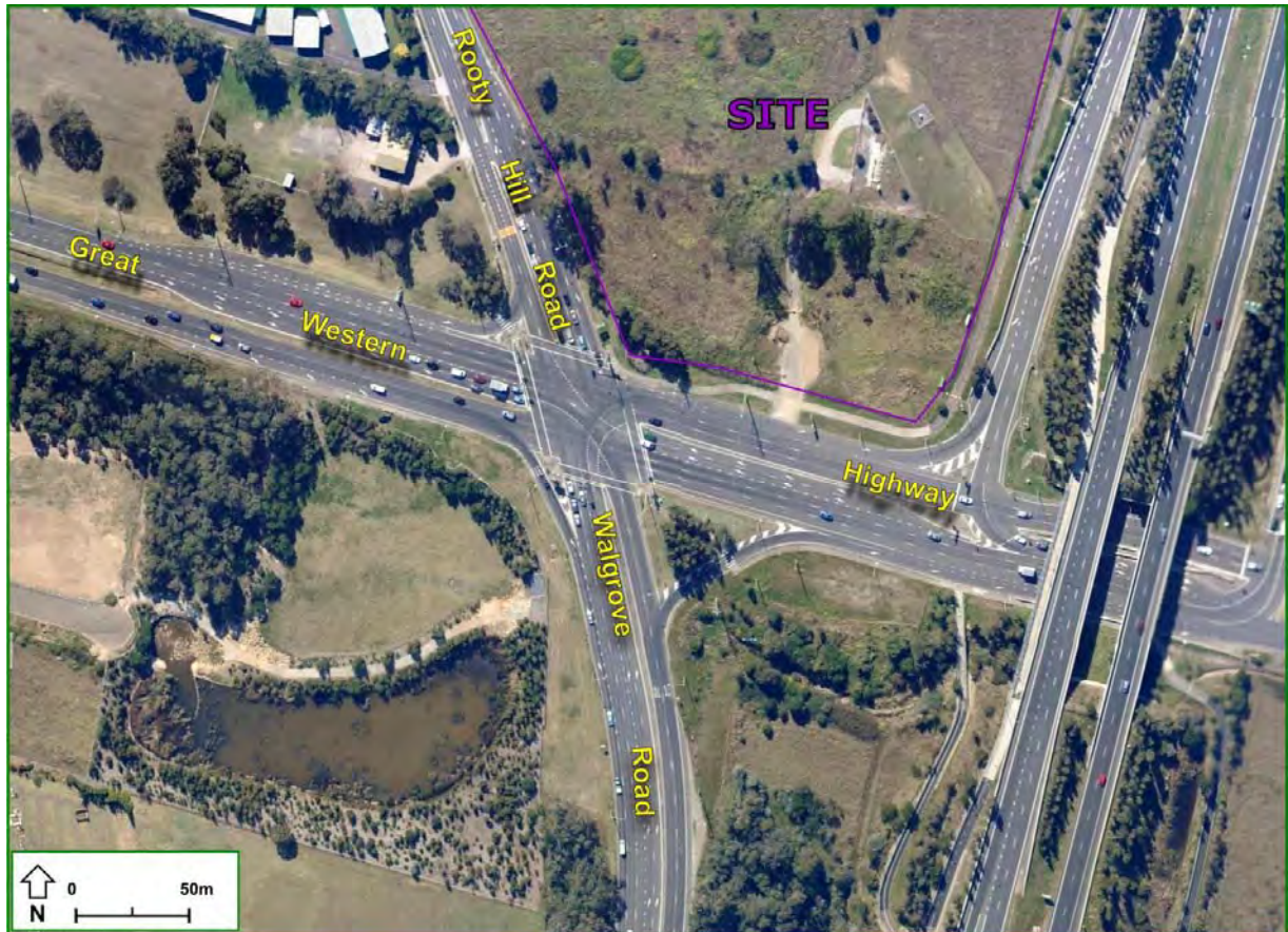
Figure 5: Intersection of the Great Western Highway with Rooty Hill Road South
