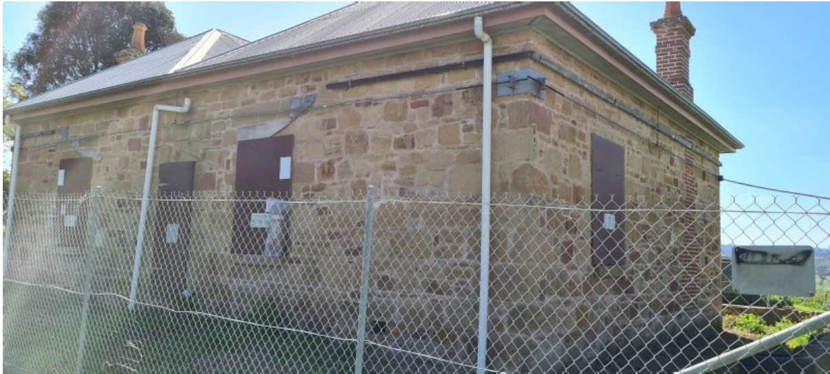
'Overdene', typical southern elevation
