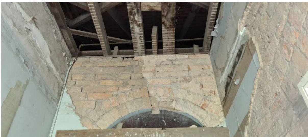
'Overdene', Internal Passage
