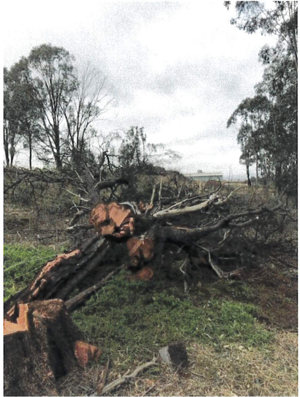
Photo 3.6 Stage 2 – clearing – post felling
