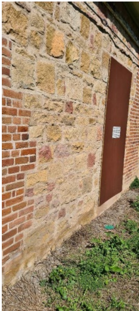
'Overdene', western elevation
