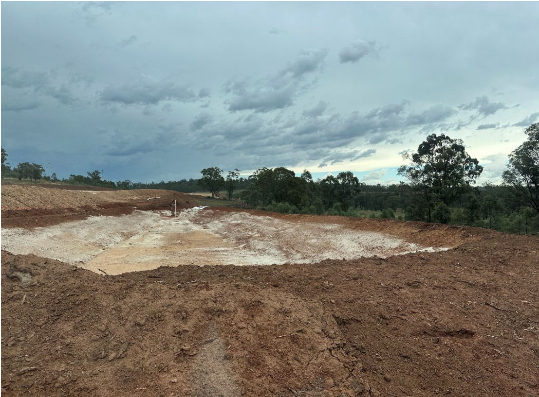
Plate 17: Erosion and sediment controls located within Western Diversion Levy Construction site (Inspection date 26/11/2025).
