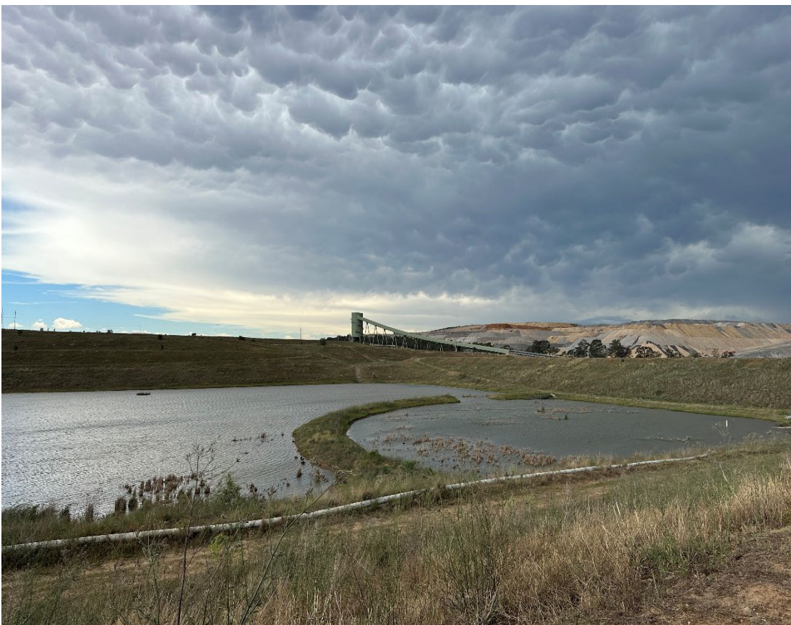
Plate 16: CW1 (Inspection date 26/11/2025).
