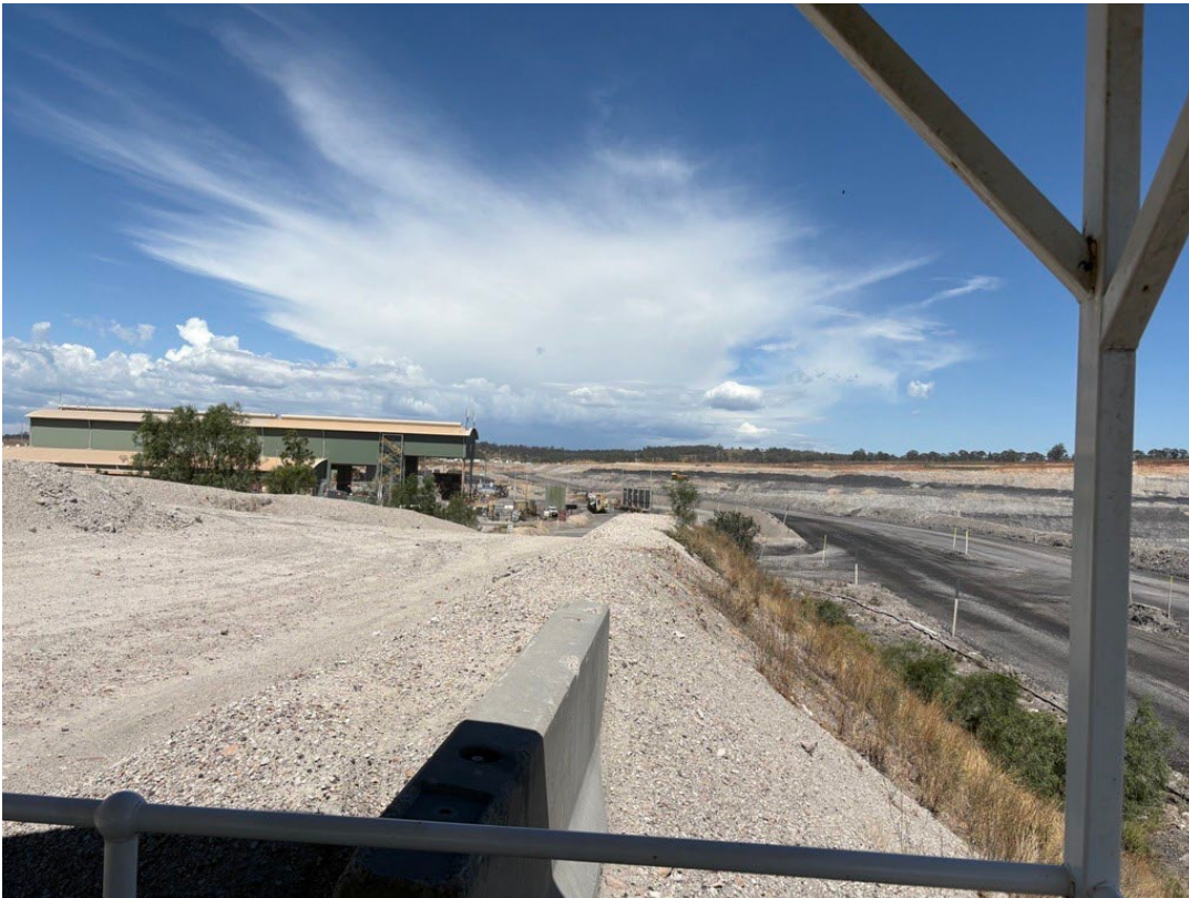
Plate 2: View from BMC viewing platform facing west. Conditions of site inspection were dry and windy, approaching stormfront (Inspection date 26/11/2025).
