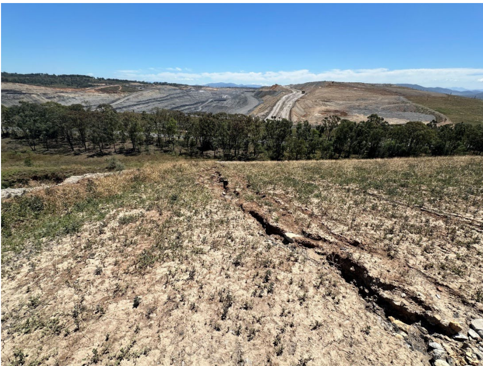
Plate 12: Rill erosion in the northern rehabilitation face. View into Mt Pleasant Mine over Wybong Road (Inspection date 26/11/2025).
