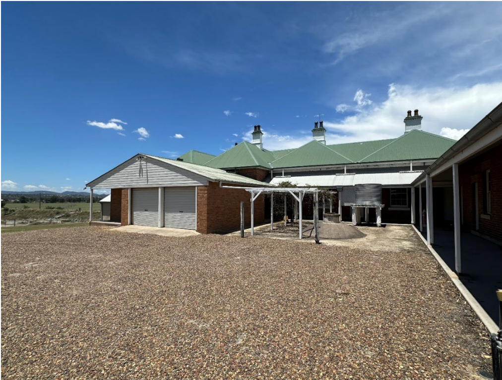
Plate 19: Bengalla Homestead (Inspection date 26/11/2025).
