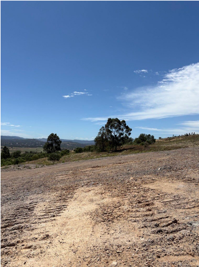
Plate 11: Old north-east rehabilitation and recently shaped rehabilitation area on the Wybong Road face (Inspection date 26/11/2025).
