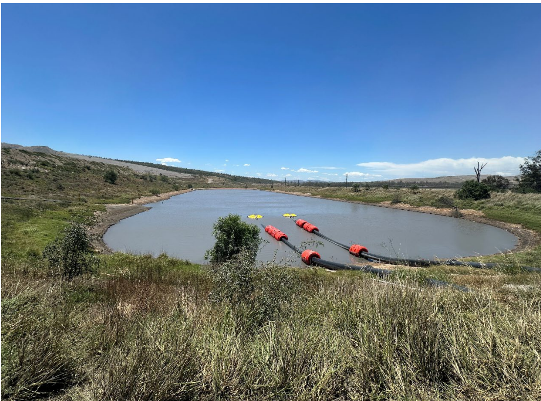
Plate 14: Dry Creek East Dam (Inspection date 26/11/2025).
