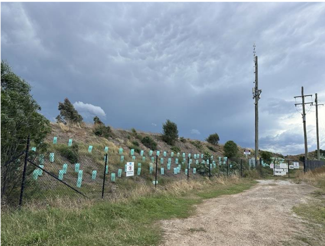
Plate 18: Earthen visual bund located along Wybong Road (Inspection date 26/11/2025).
