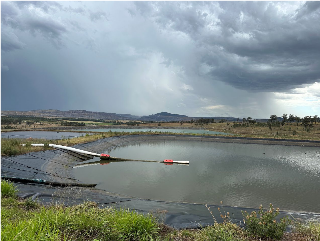
Plate 15: Hunter River Raw Water Dam (Inspection date 26/11/2025).
