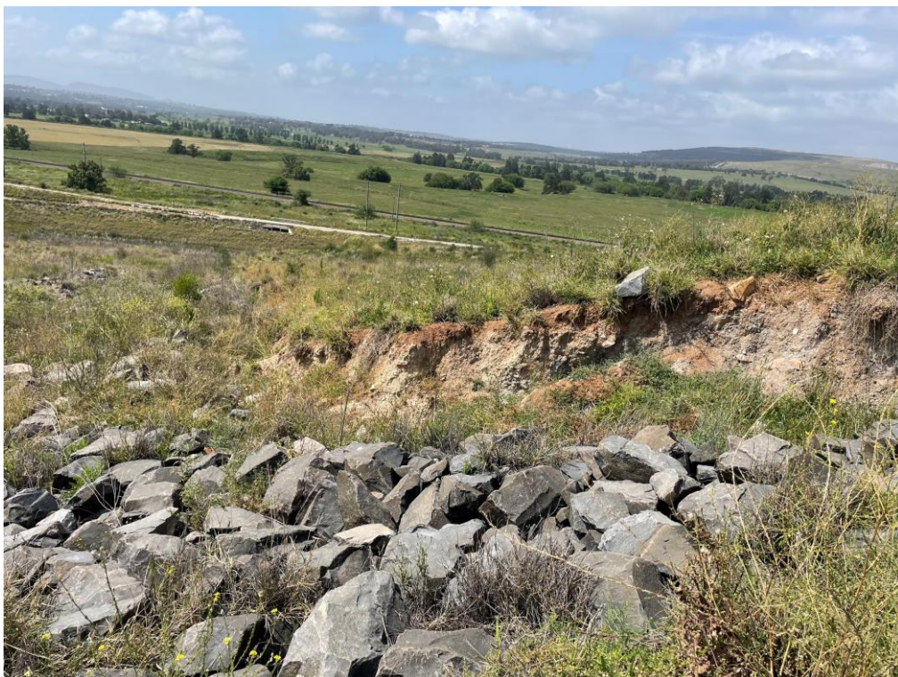
Photo 7 – Moderate scour erosion in drain in Zone 2
