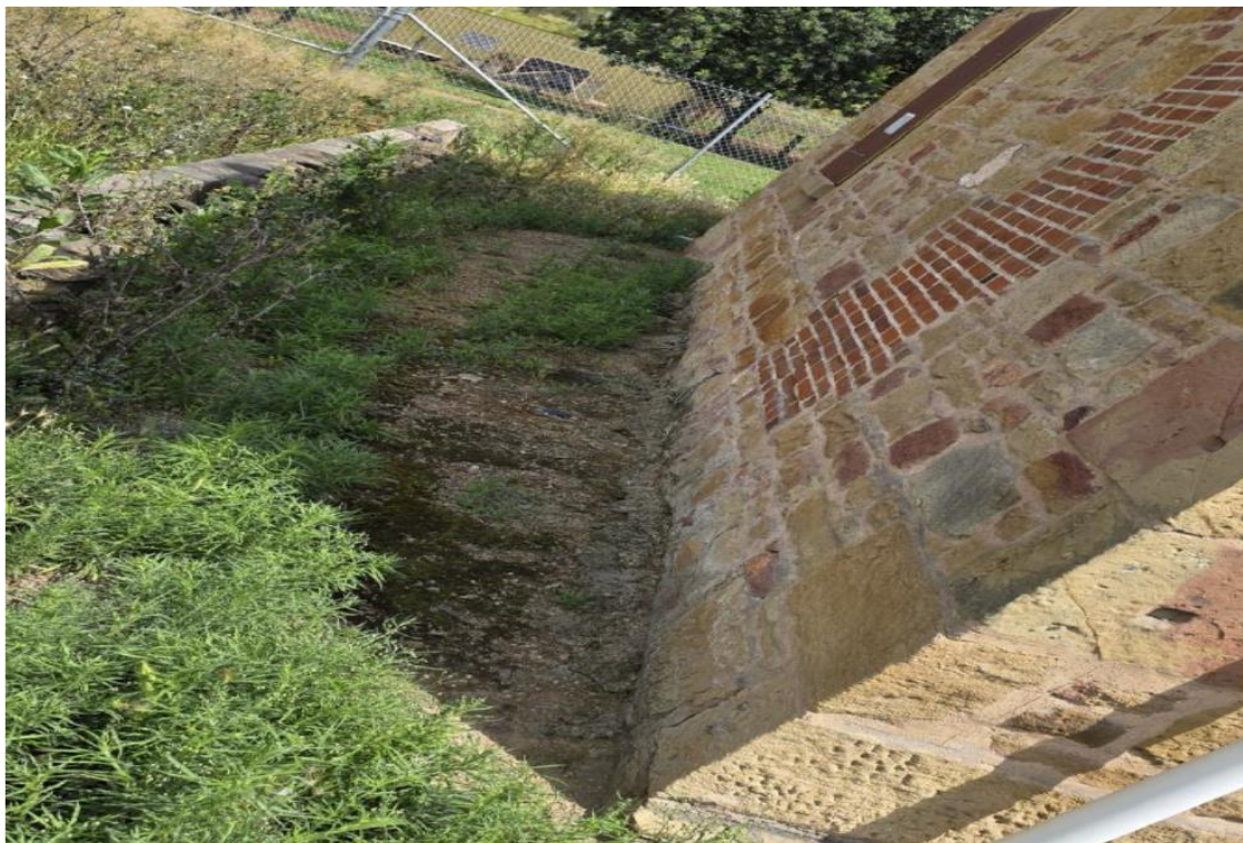
External view of exposed verandah area
