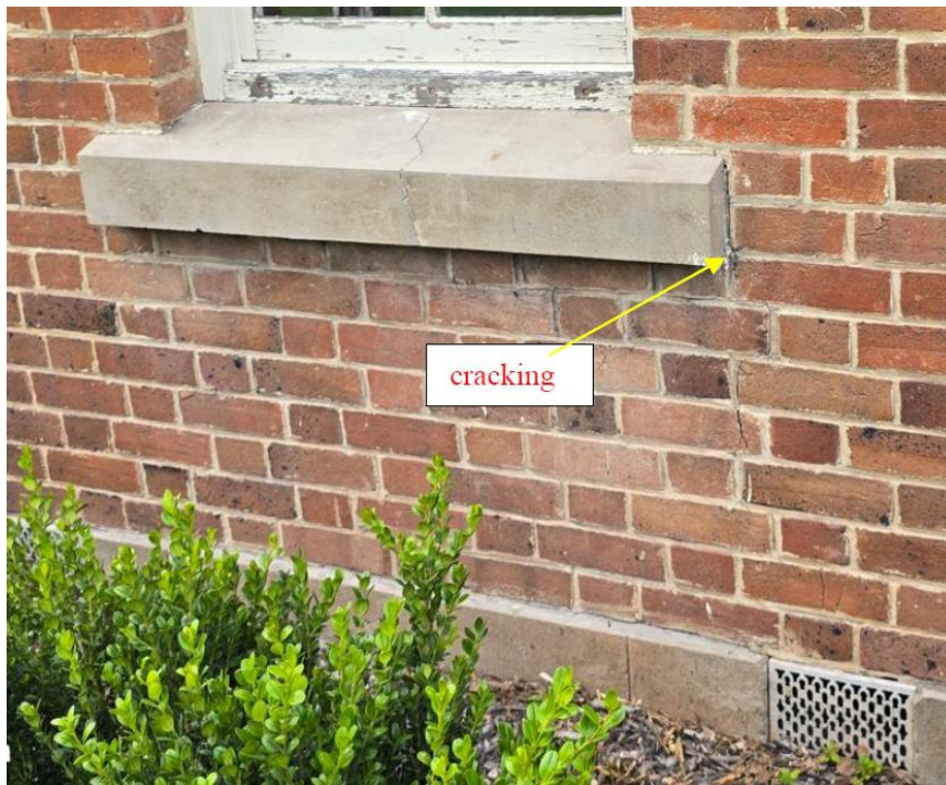
Example of brick and mortar repairs needed
