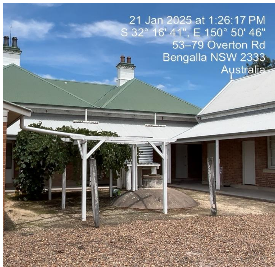
Main homestead, northern aspect
