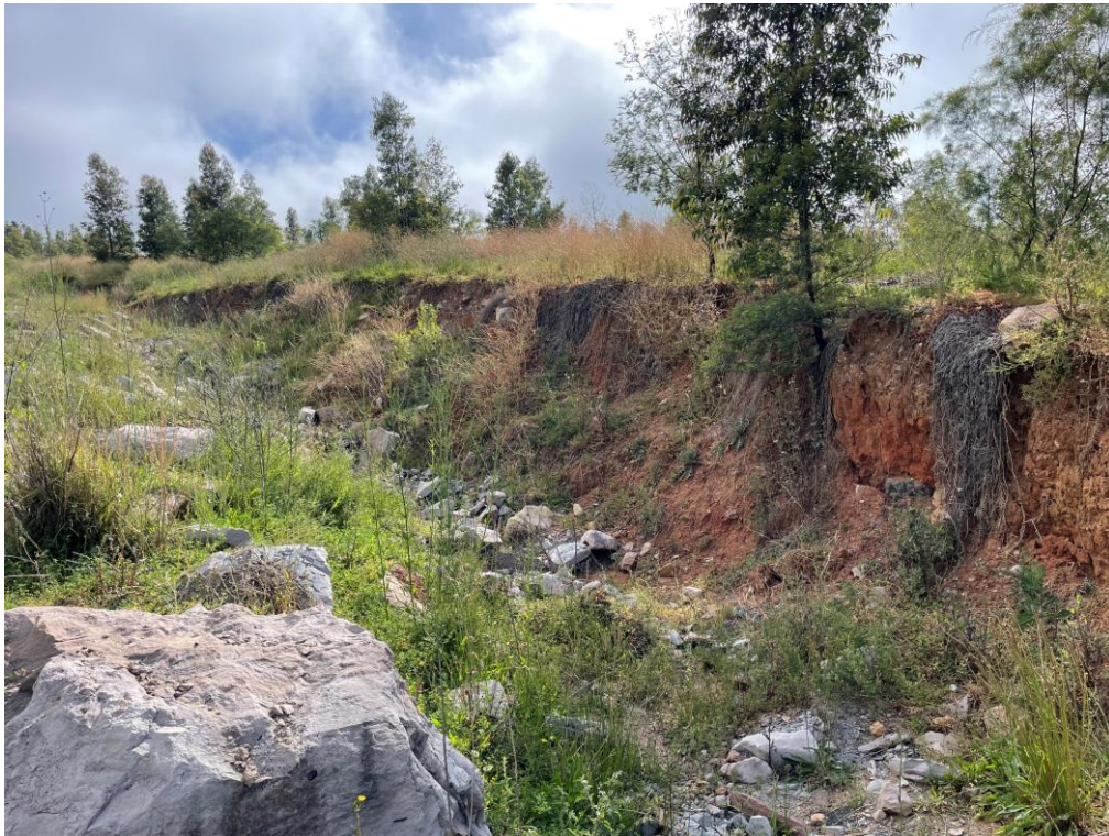
Photo 7 – Moderate scour erosion in drain in Zone 2
