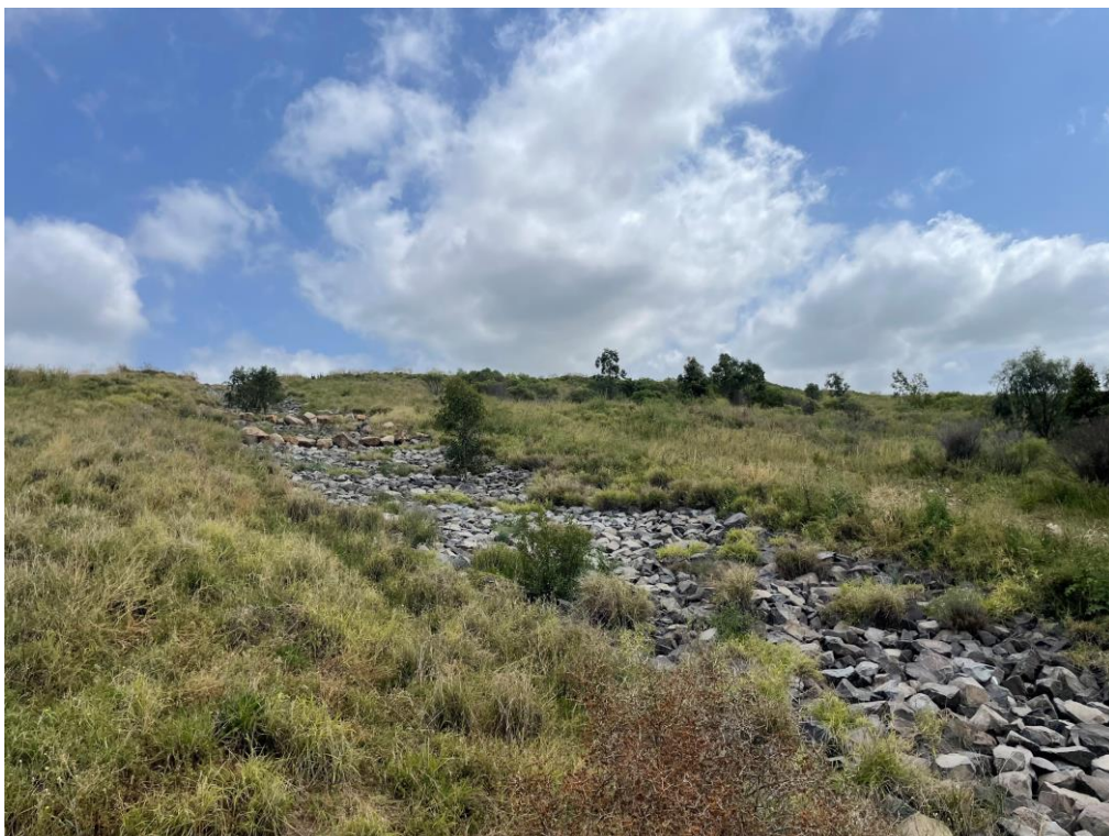
Photo 9 – Example of stable and vegetated drop structure
