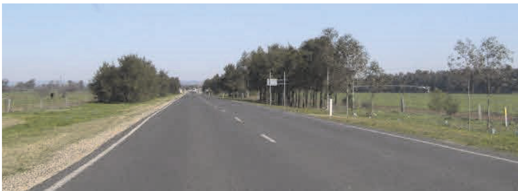
Figure 3 Bengalla Link Road, looking northbound from north of Wantana Dairy.
