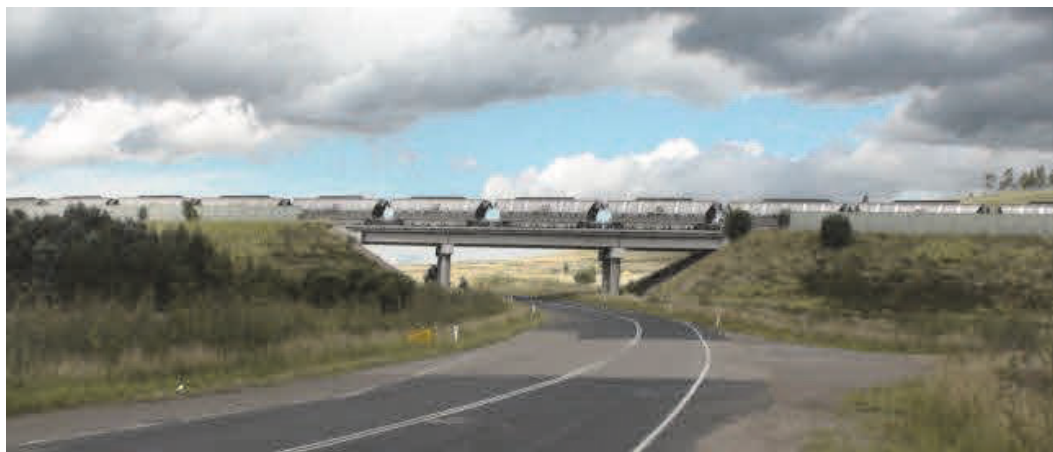
Figure 6 Thomas Mitchell Drive, looking southbound towards the Antienne Rail Spur (MAC rail overbridge)
