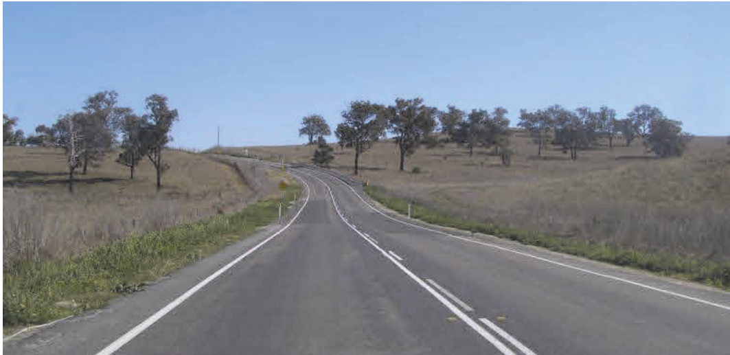
Figure 4 Wybong Road, west of Spring Creek (looking west).
