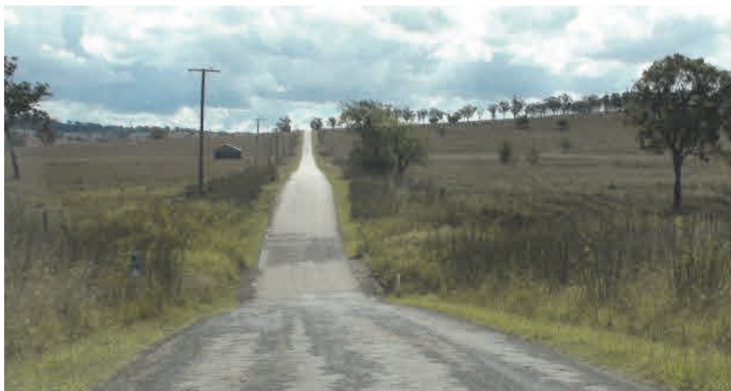
Figure 5 Edderton Road, looking north towards the Saddlers Creek floodway
