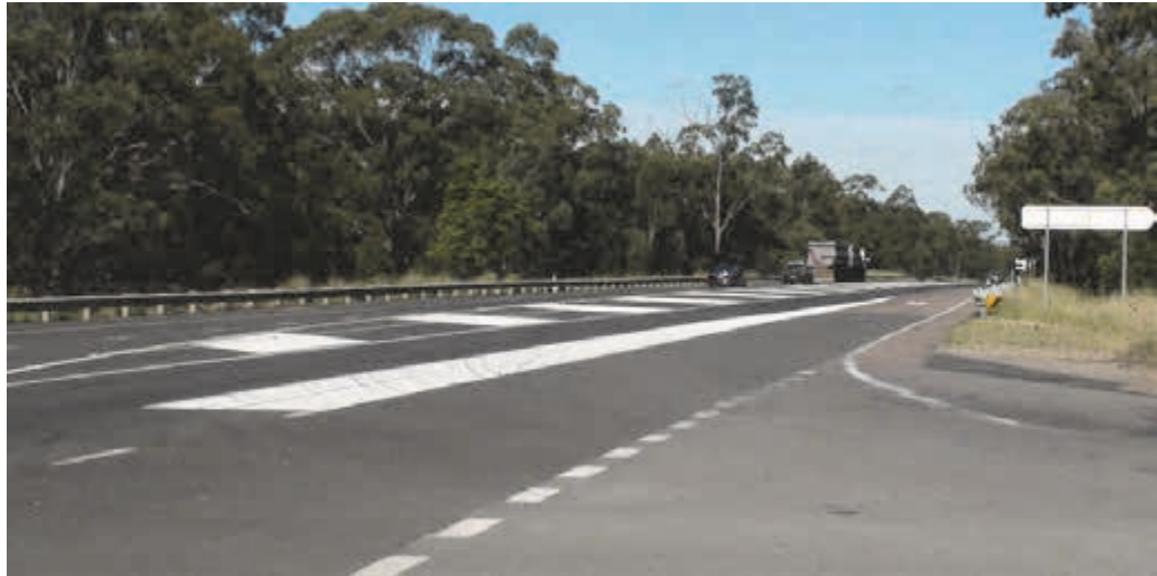
Figure 13 Looking south from the Thomas Mitchell Drive hold line towards the New England Highway.
