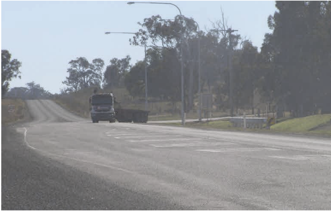
Figure 10 Bengalla Link Road, looking northbound towards the intersection with Bengalla Mine Access Road (right-hand side)
