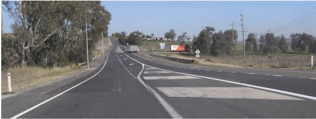
Figure 11 Denman Road looking westbound towards the intersection with Bengalla Link Road (right-hand side).
