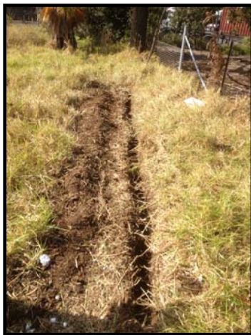
Length of trench 6 x metres to 600mm in depth at a setback of 3.6 metres from the tree trunk centre
