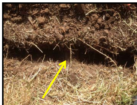
1 x root encountered (130mm) offset 2.5 metres to the east of trunk centre 100mm below grade
