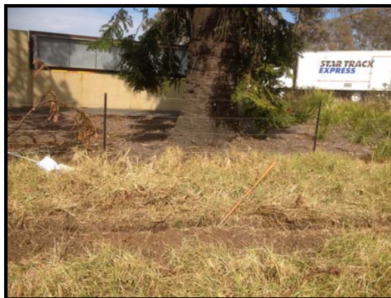
Length of trench 6 x metres to 600mm in depth at a setback of 3.6 metres from the tree trunk centre
