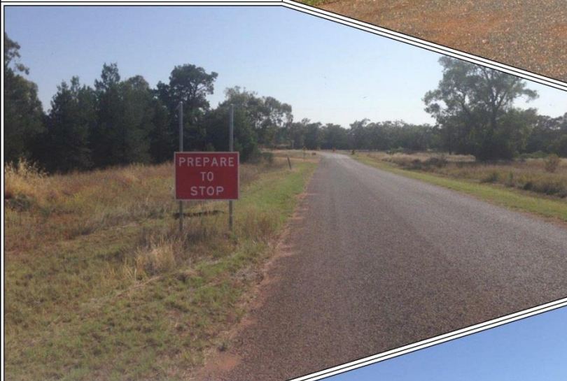
Plate 2.3: View of Gilgai Road looking northeast (Source - Constructive Solutions (2016) - Plate 3)
