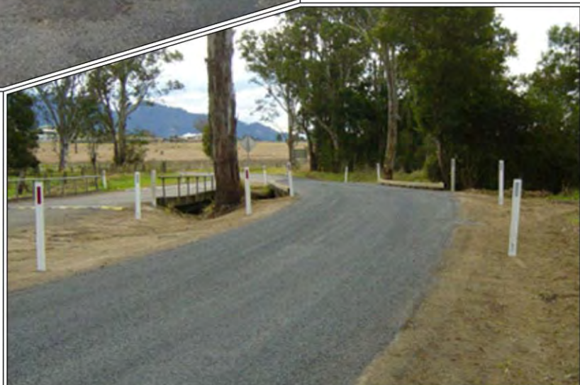
Plate 4.8: Fairbairns Road - bridges over Avon River. (Ref: Constructive Solutions 2016 - Plate 10)
