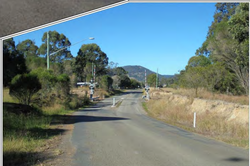
Plate 4.4: Rail Crossing of Jacks Road - Looking East. (Ref: Constructive Solutions 2016 - Plate 29)
