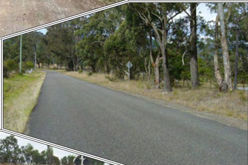
Plate 4.6: Fairbairns Road - typical alignment and condition. (Ref: Constructive Solutions 2016 - Plate 8)
