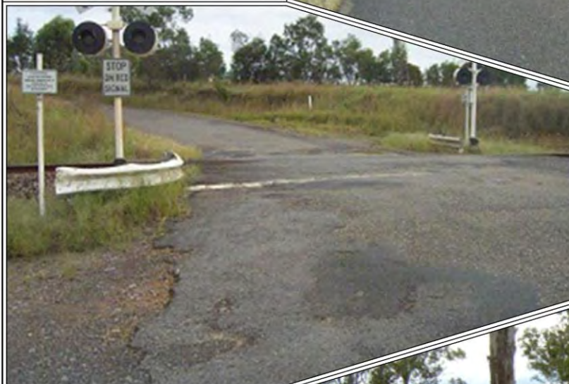
Plate 4.7: Fairbairns Road Rail Crossing - looking west. (Ref: Constructive Solutions 2016 - Plate 30)
