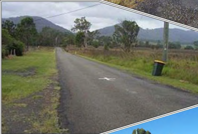
Plate 4.3: Jacks Road - typical alignment and condition. (Ref: Constructive Solutions 2016 - Plate 5)
