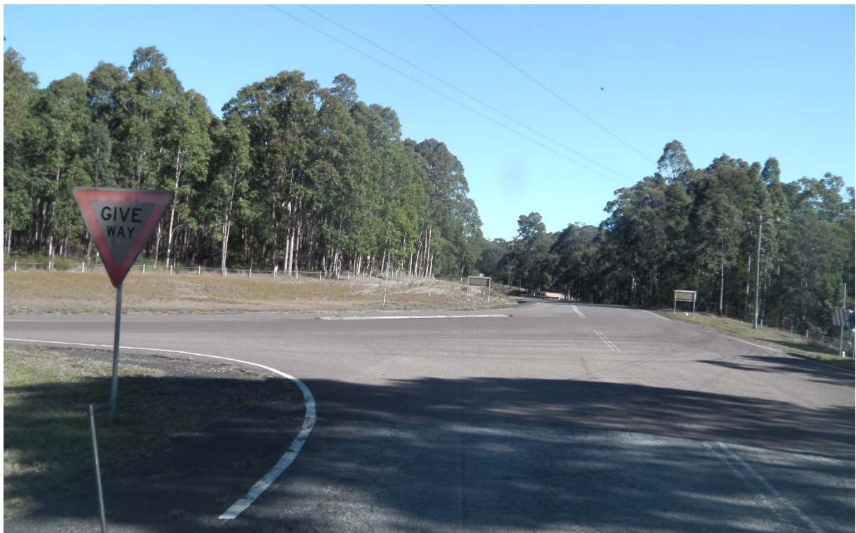
At the intersection looking south
