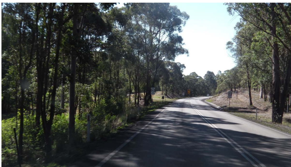
Approach to the intersection looking north
