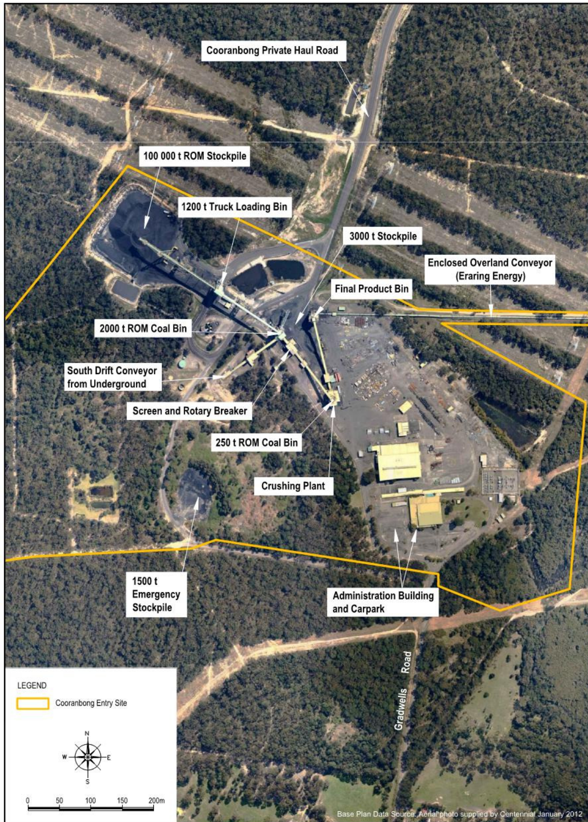
Figure 4: Mandalong Mine - Cooranbong Entry Site
