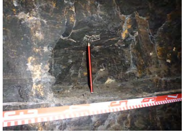
Plate 2 View of cut groove and ventilation shaft (Bat Alley)
