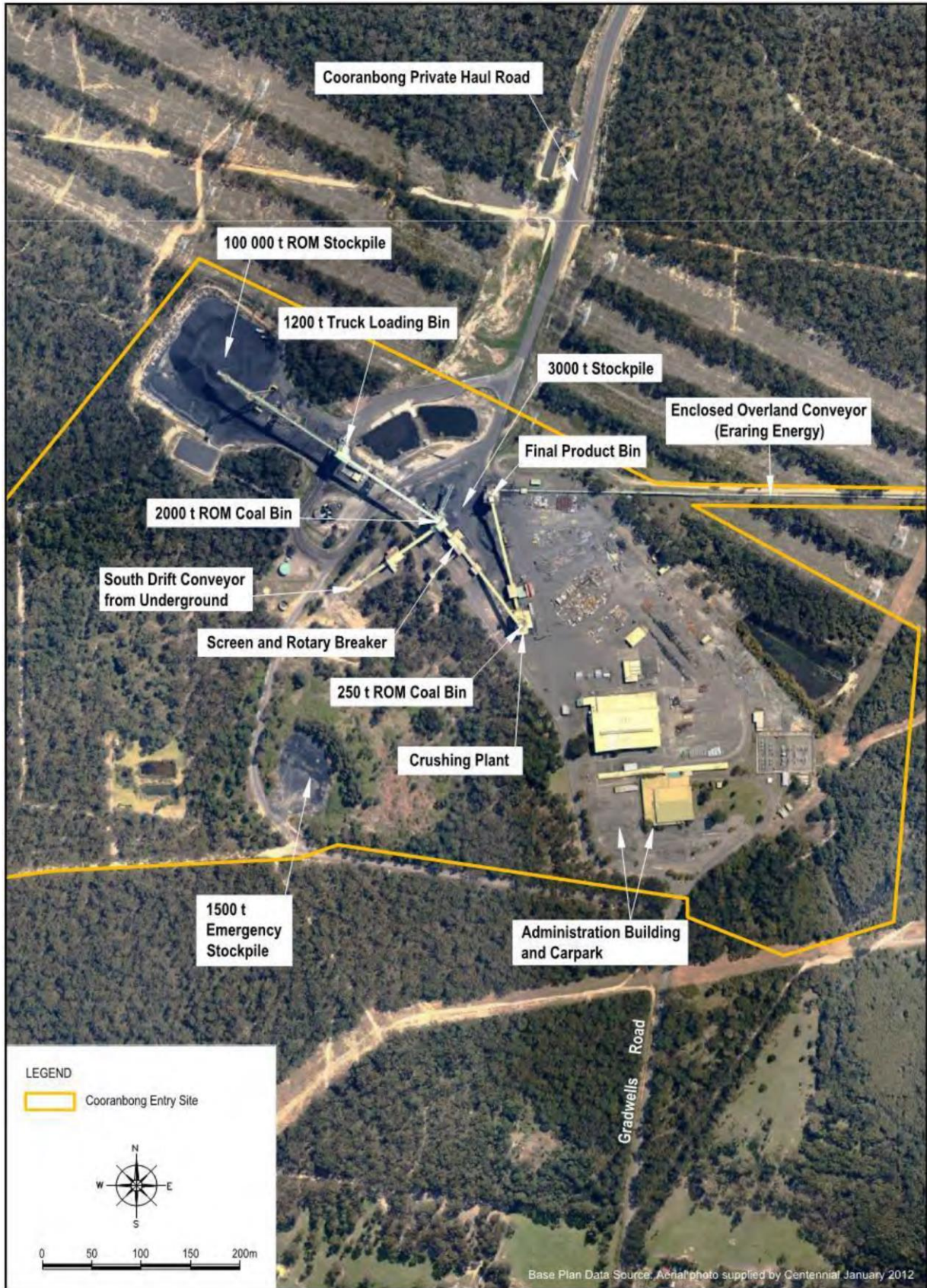
Figure 2: Cooranbong Entry Site (CES)
