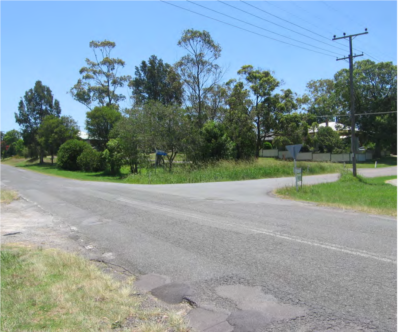
Photograph 6 – Newport Road / Gradwells Road intersection, Dora Creek
