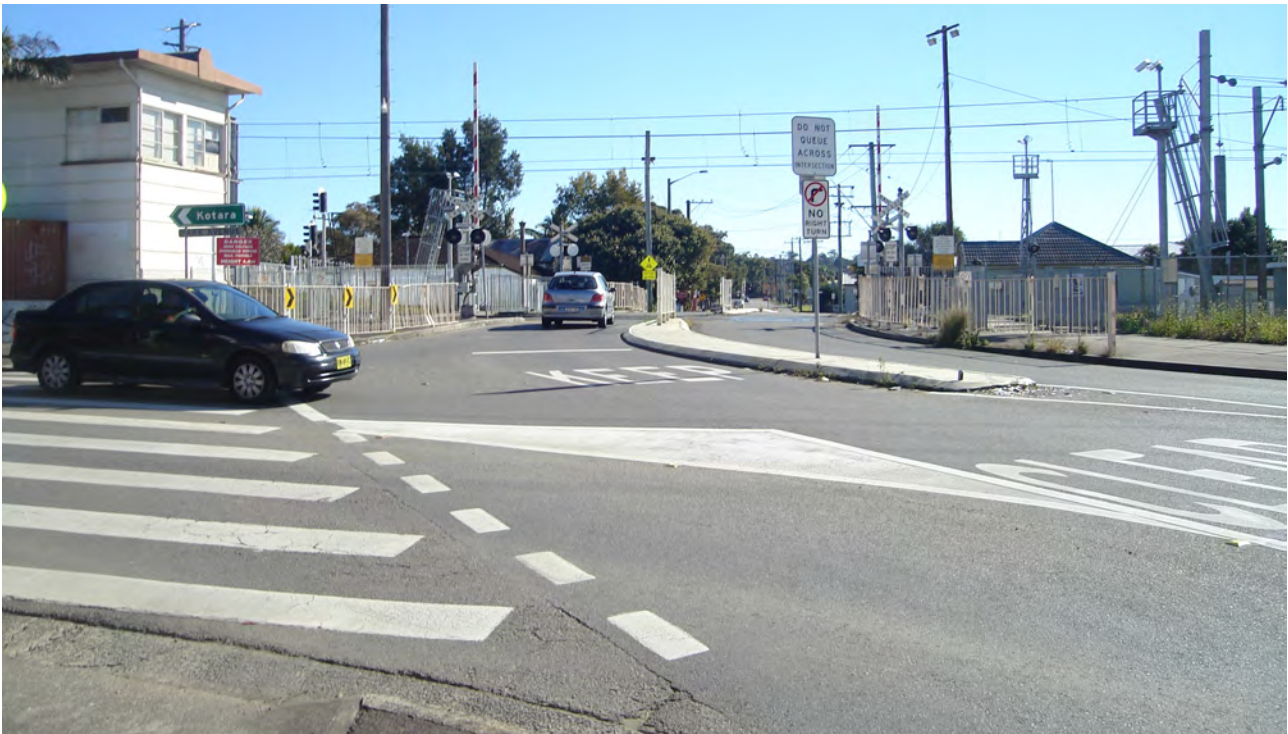
Photograph 7 – Glebe Road, Adamstown level rail crossing
