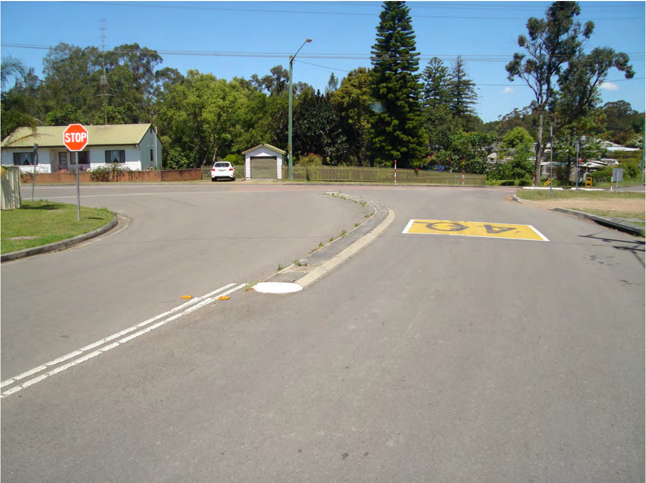
Photograph 3 – Miller Road / Macquarie Road intersection
