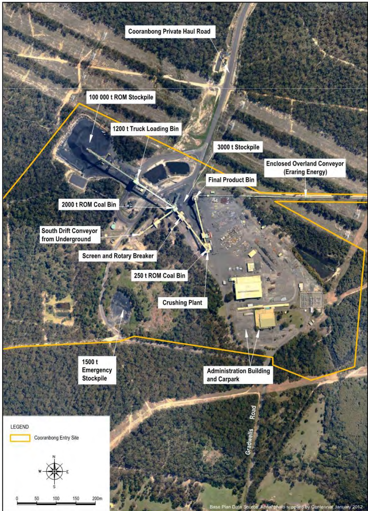
Figure 4 Mandalong Mine - Cooranbong Entry Site
