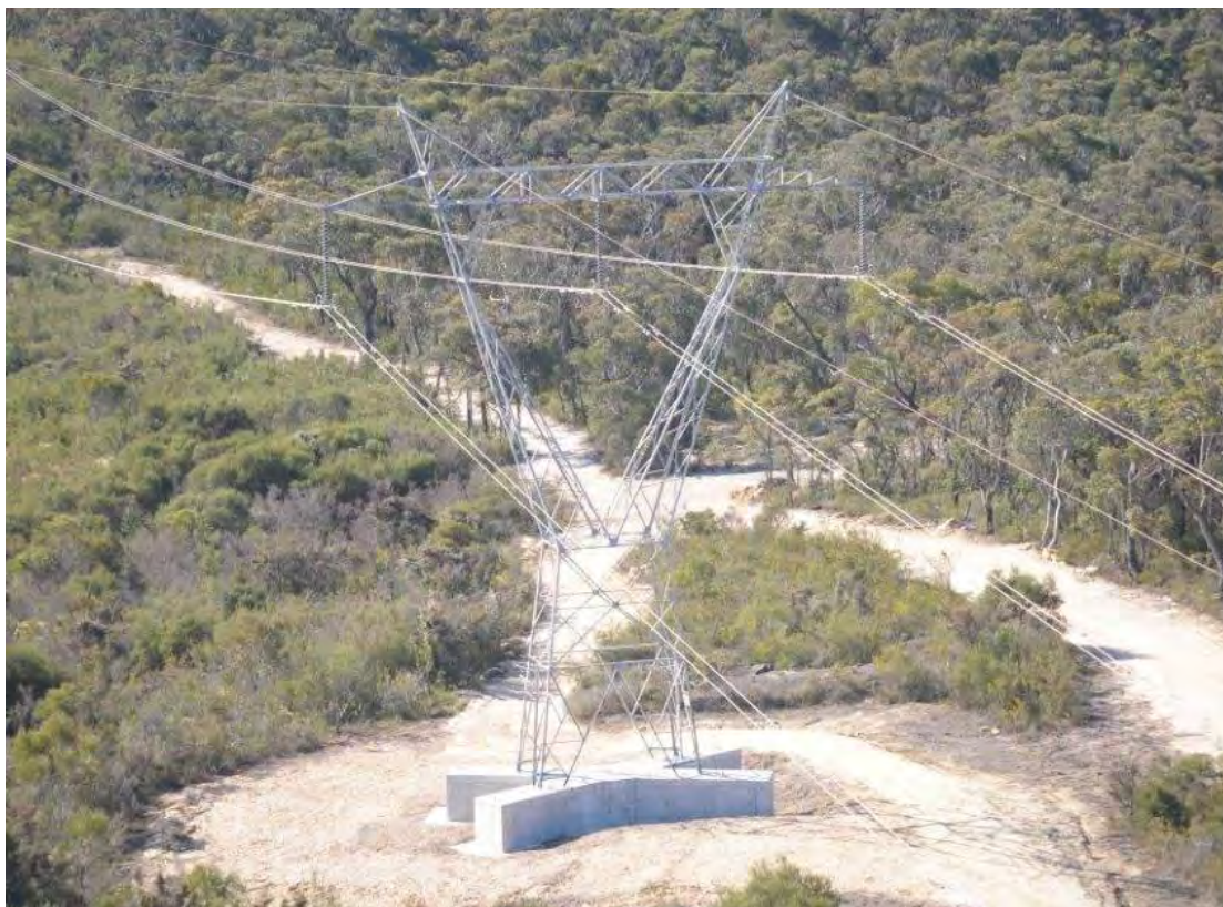
Figure 2: Example of structure with completed cruciform foundation
