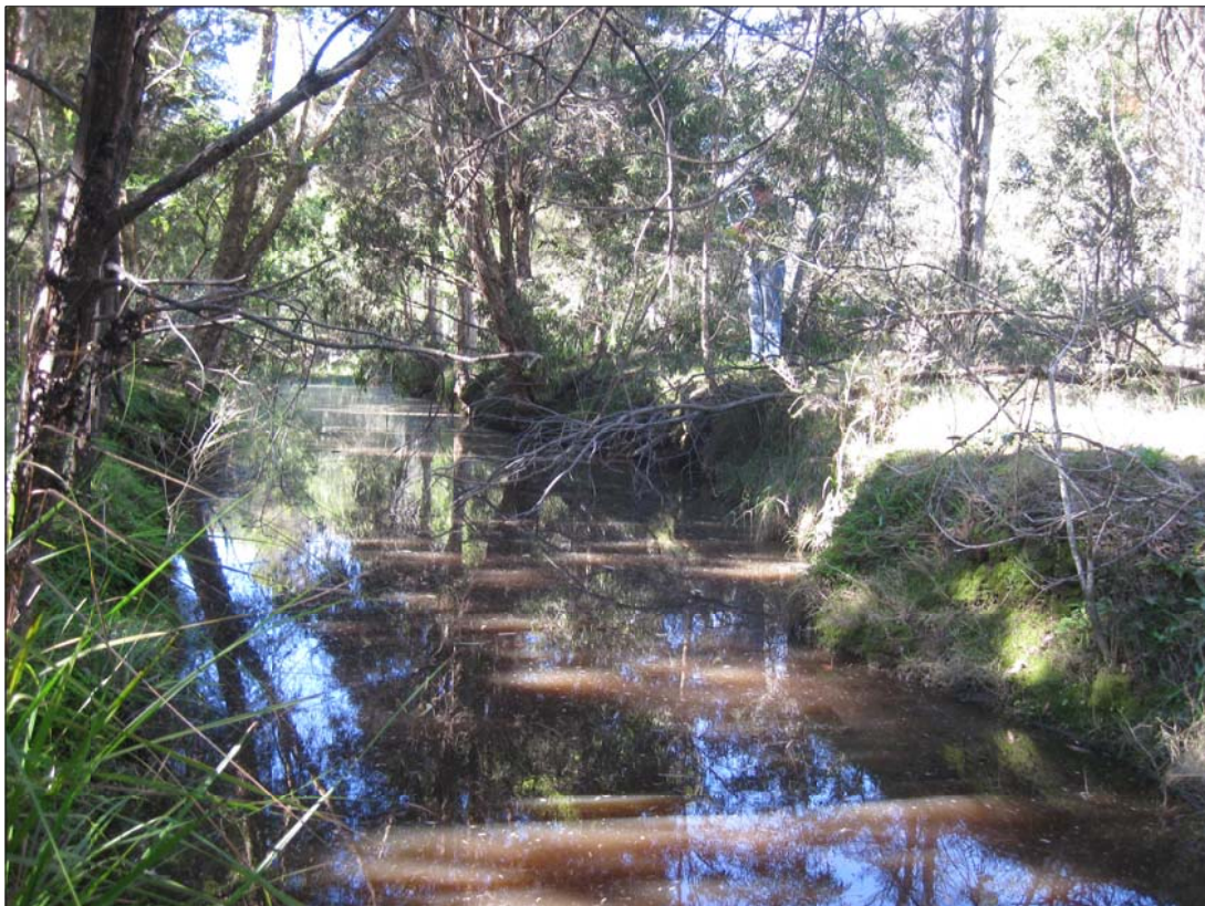
PLATE 3.6 Scouring within Lower Catchment Area of Wyee Creek, Looking Downstream from Schofield Road (June 2011)
