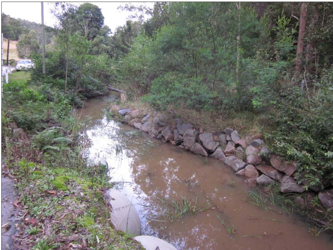
PLATE 3.4 Bank Stabilisation Works within Wyee Creek, Looking Downstream from Wyee Farms Road (June 2012)
