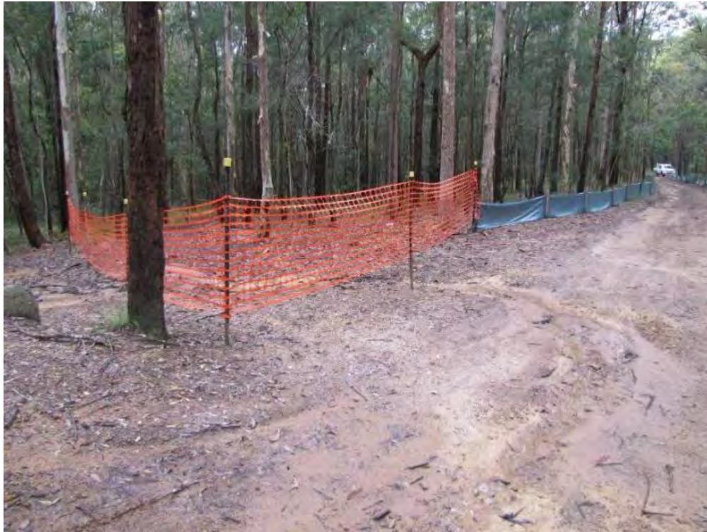
Plate 35 High visibility fencing and silt– recommended
