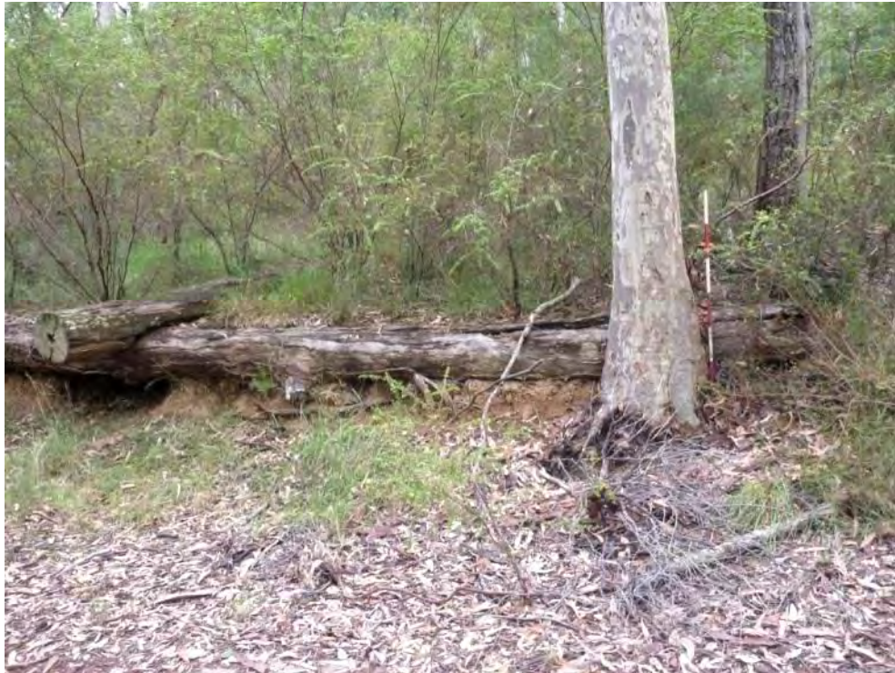
Plate 39 Landing Skid 2 - elevation from track, note live tree right hand side as support for structure
