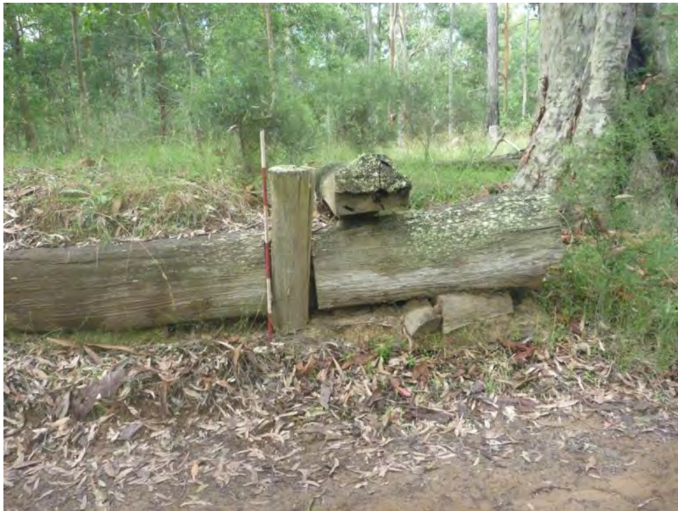
Plate 44 Landing Skid 4 - From track showing underside of skid which has been sawn flat
