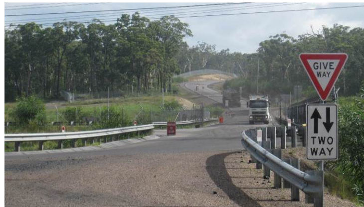
Plate 8 – Start of the Private Haul Route at the Cooranbong Entry Site
