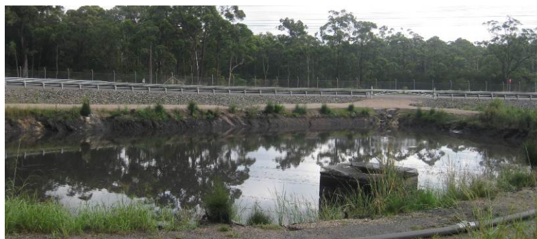
Plate 10 – Sediment Dam at Cooranbong Entry Site
