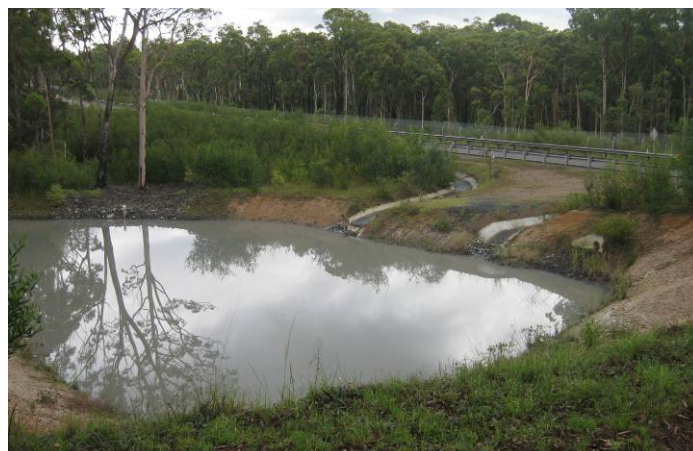
Plate 11 – Sediment Basin along Private Haul Road
