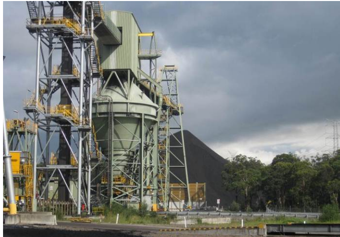
Plate 7 – Truck Loading Bin and Coal Stockpile
