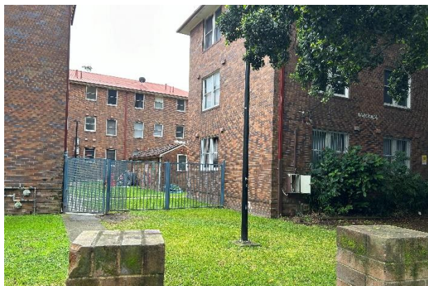
Figure 7 Residential flat buildings to the north of Kettle Street
