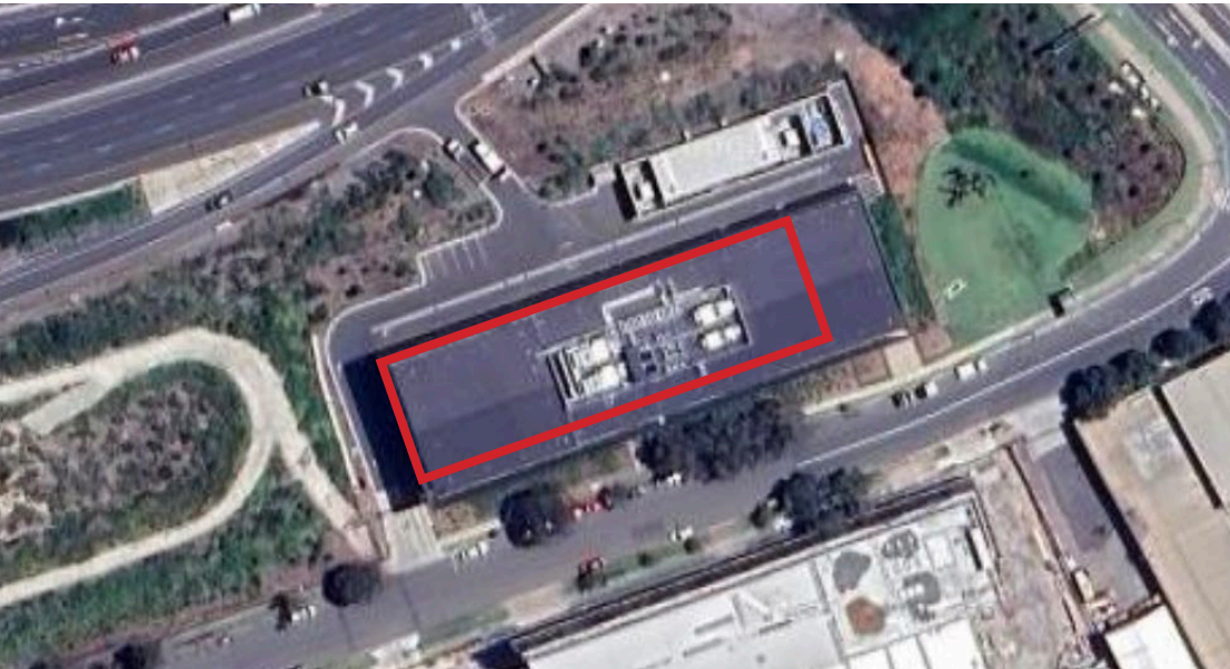
WestConnex Control Centre, S1 scale comparison
