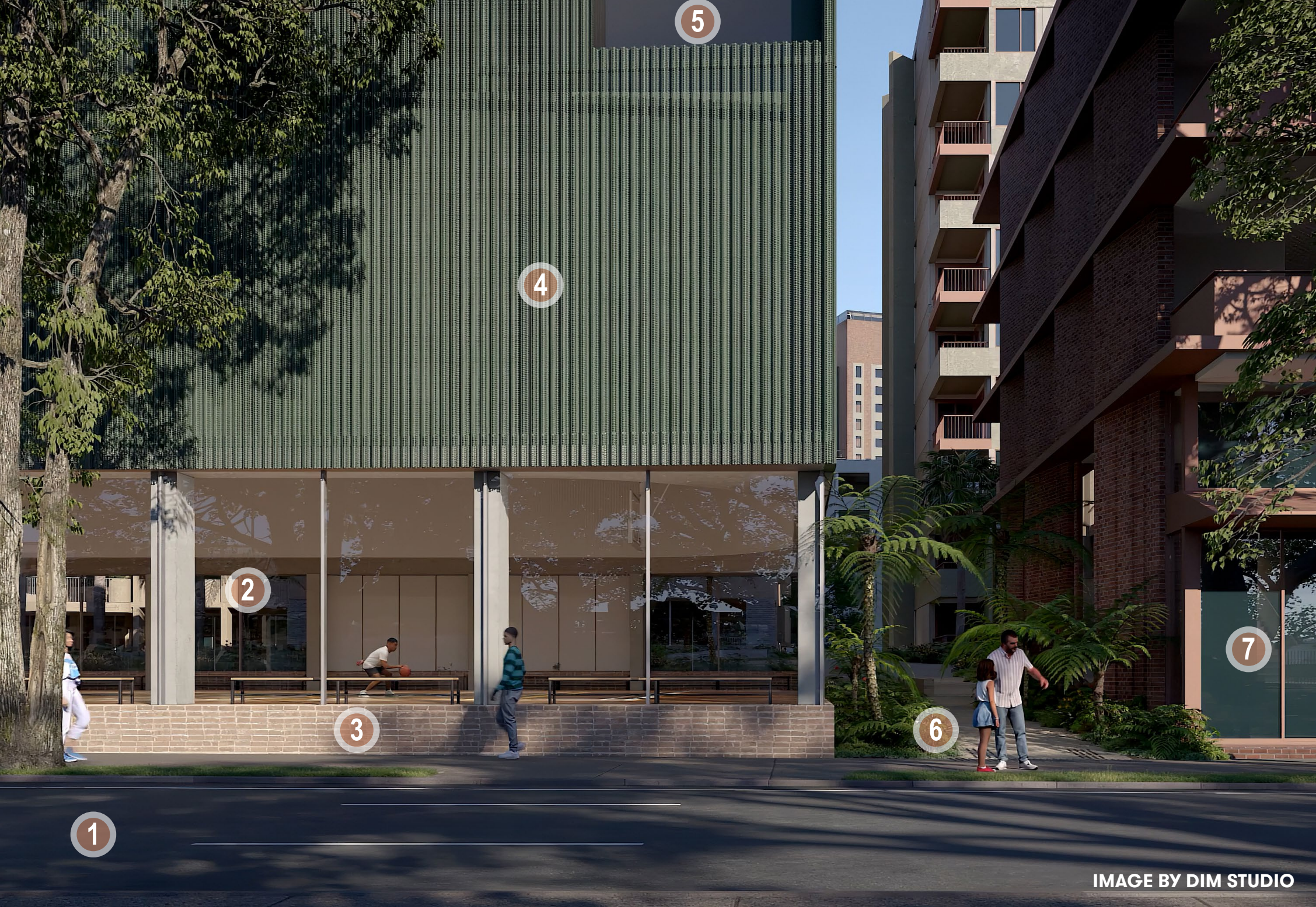
Western facade viewed from Elizabeth Street facing east.
