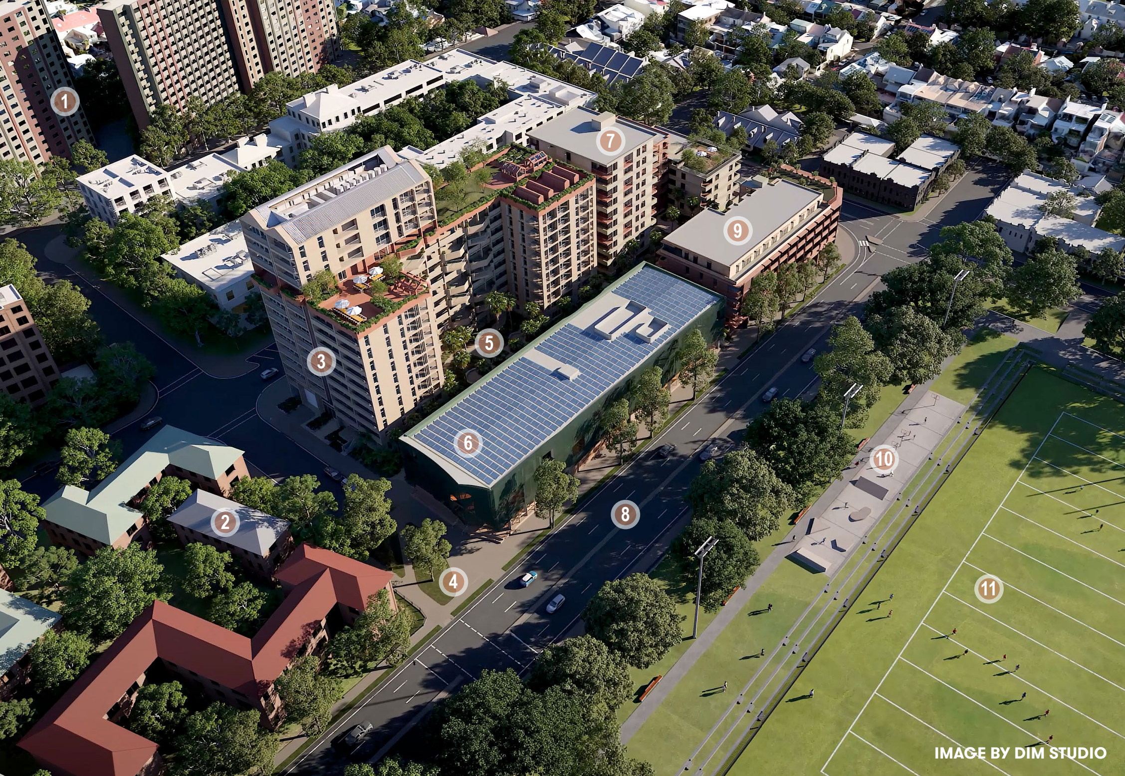
Aerial view from the north west showing the proposed precinct including S1, S2, S3 & S4.
