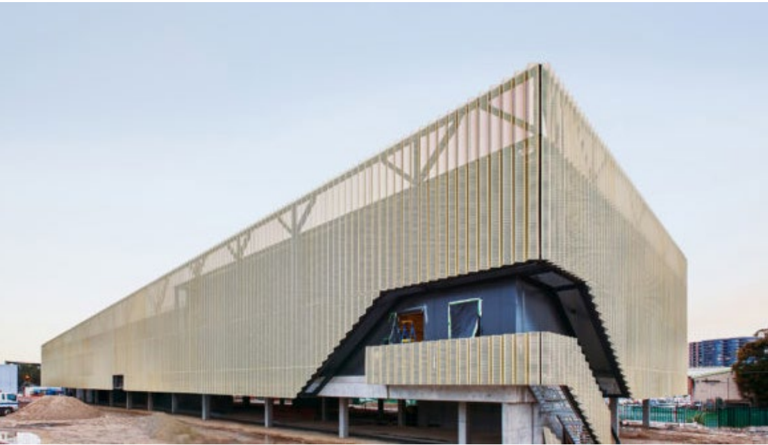
WestConnex Control Centre
