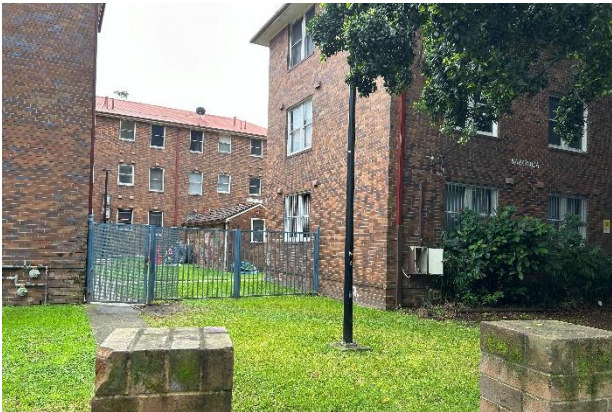
Residential flat buildings to the north of Kettle Street
