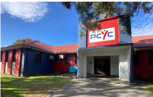
Existing PCYC Building
