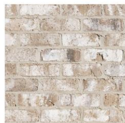
4. Face brickwork, colour matched mortar
