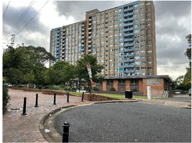
Figure 10 Residential apartments on Morehead Street
