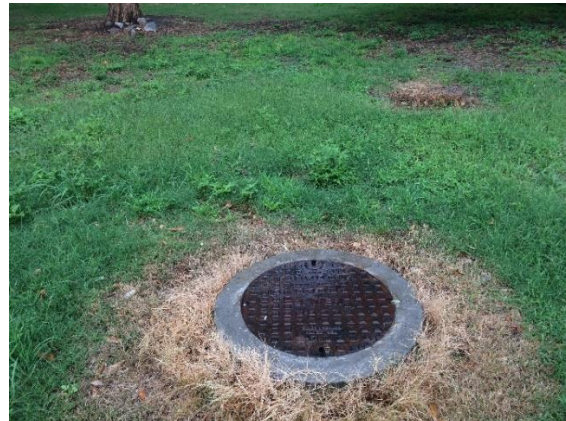
Figure 28. Sewer manhole in centre of subject area.
