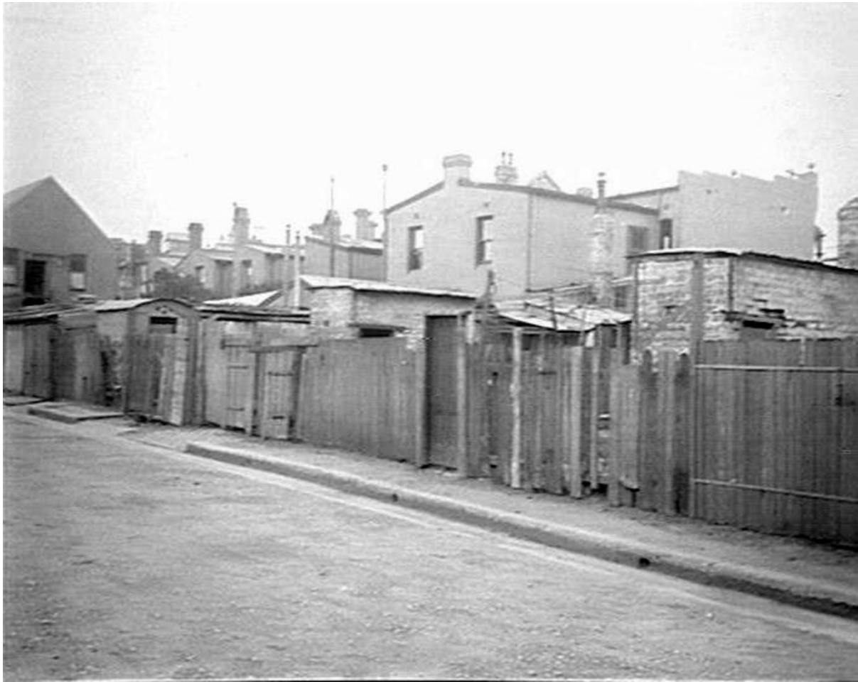
Figure 13: Alderson Street showing backyards, date unknown, however Alderson Street was formed only during the late nineteenth century period of subdivision (Source: SLNSW Government Printing Office 1 – 31164).
