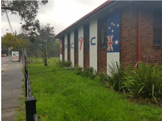
Figure 25. Entry to the PCYC building in the southern portion of the site, view north.
