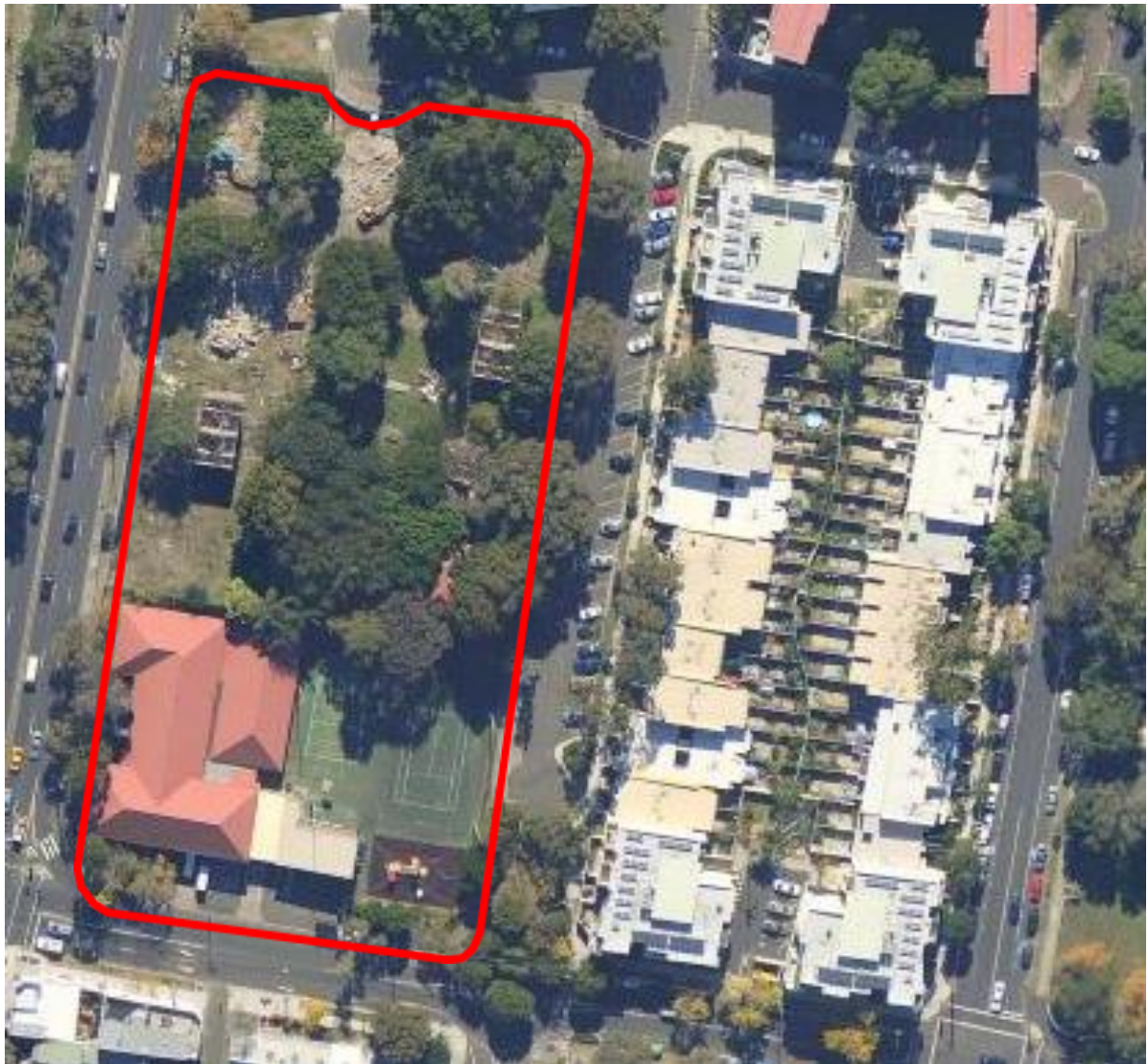
Figure 24. Nearmaps imagery May 2013 showing structures being demolished, the site is now vacant except for the large mature trees and the remaining PCYC building.
