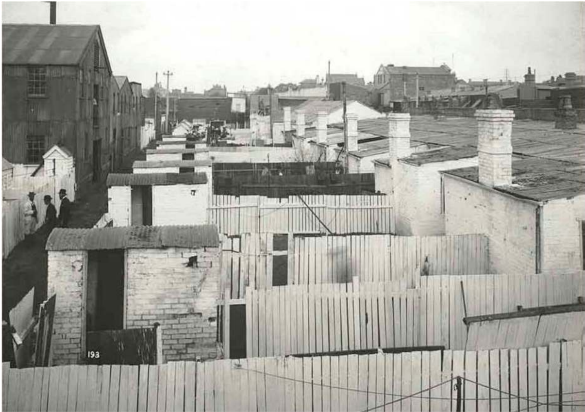
Figure 7. Rear of Alderson Street, Sydney (Redfern), about 1900. Source: State Records of NSW, NRS 12487, Digital ID: 12478_a021_a021000048.
