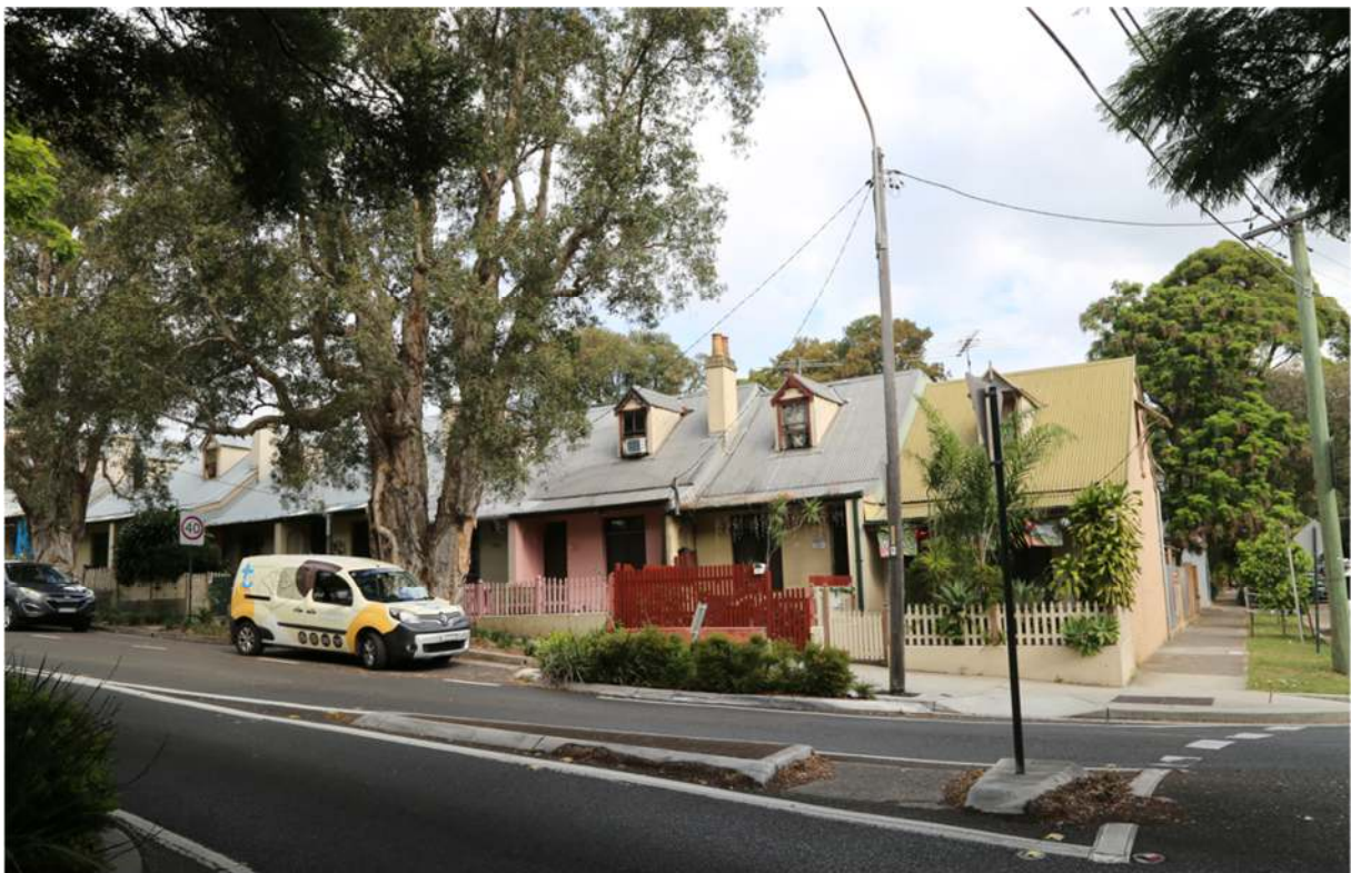
Figure 25. View of terrace housing on Phillip Street which forms part of the Waterloo HCA.
