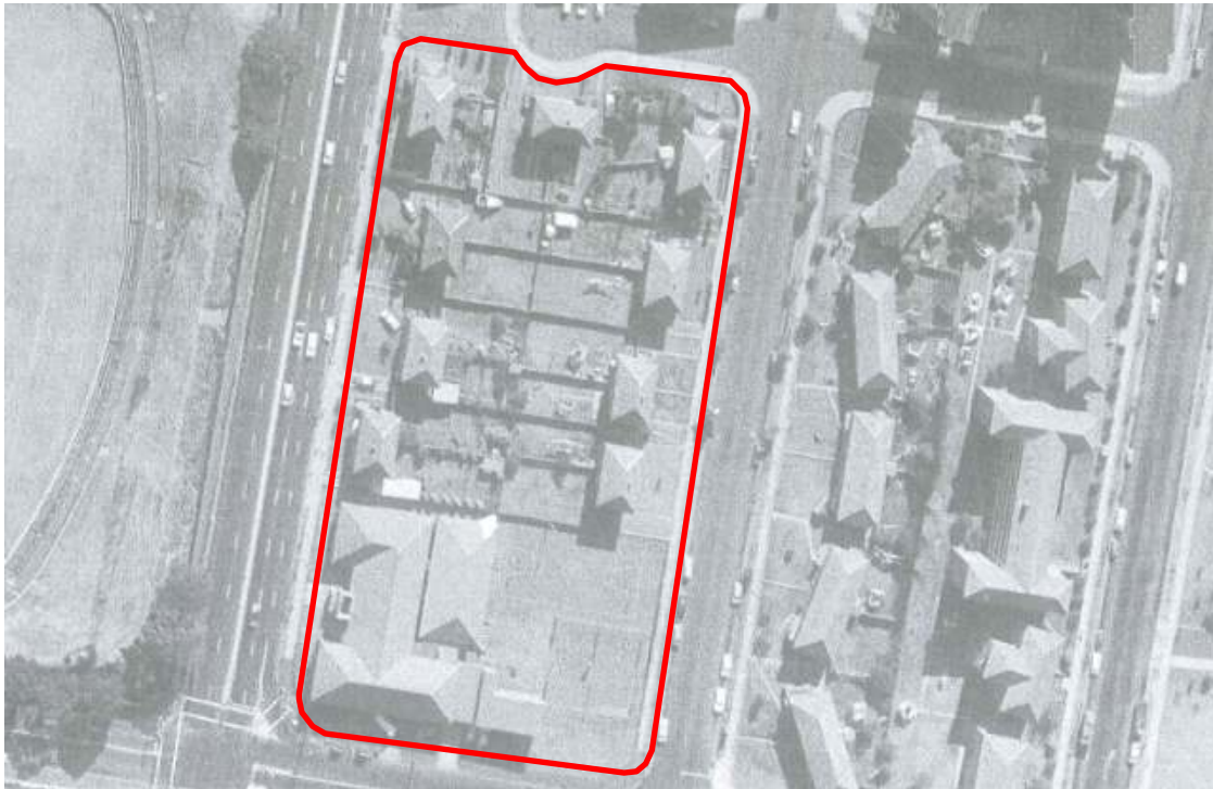
Figure 12. 1970 aerial photograph of the subject site. Source: Land and Property Information, Cumberland Survey Run 18, 07.07.1970, Map 1909_5102.
