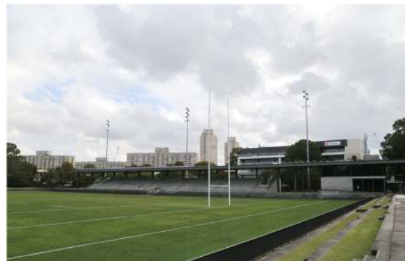
Figure 17. View from Redfern Oval facing Waterloo Social housing development in the background.
