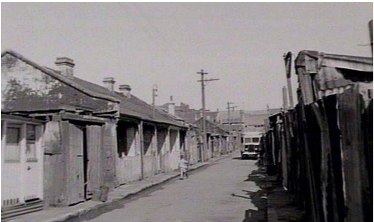
Figure 6. Redfern Slum Dwellings like those in the subject site, slated for demolition. Source: SLNSW Government Printing Office 2 – 03527, in Extent/AHMS 2014: 52.
