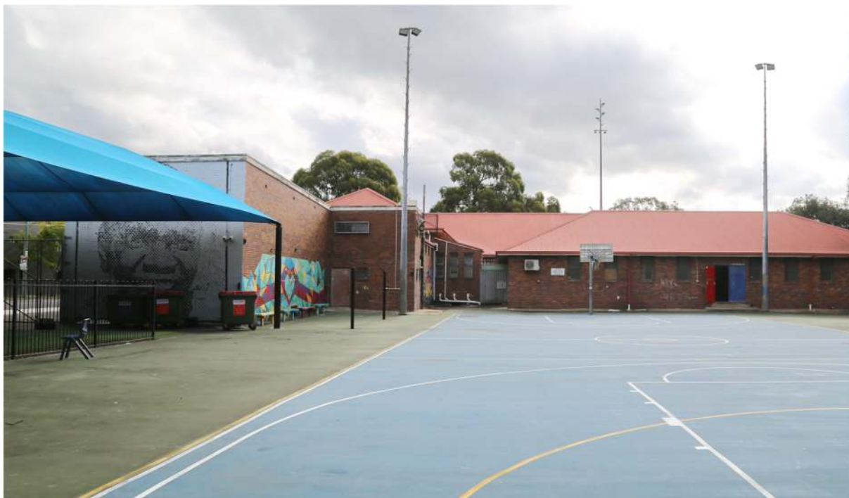
Figure 29. View from basketball court facing west to the rear of the PCYC buildings.
