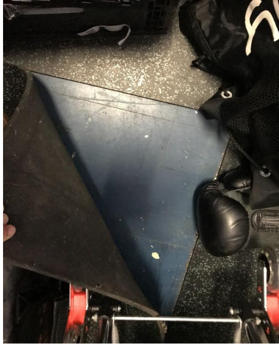
Photograph 3: PCYC, interior, stationary store, floor, below matting - blue vinyl floor tiles.
