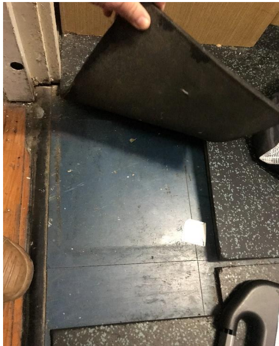
Photograph 4: PCYC, interior, stationary store, floor, below matting - blue vinyl floor tiles.
