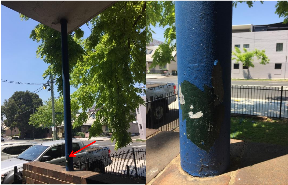
Photograph 19: PCYC, exterior, southern façade, western awning, metal supports posts, typical blue and underlying green paint, lead paint (>0.1% lead w/w)
