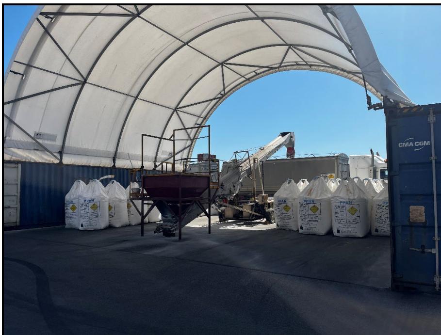
Photo 16: AN unloading shelter with bulka-bags of AN being unloaded via conveyor into a truck. Looking to the north.
