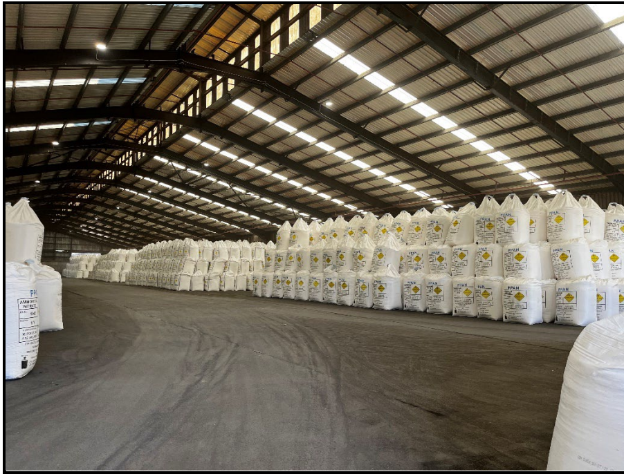
Photo 13: View inside Shed B from the door. Looking to the west.
