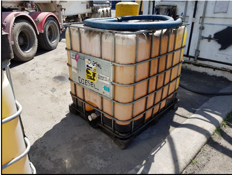
Photo 9: IBC labelled as containing Diesel located in the bund for the refuelling area.
