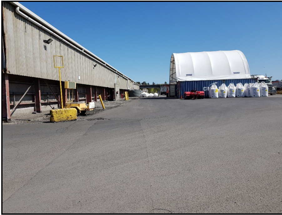
Photo 15: View to the west and the AN unloading shelter, Shed A on the left.
