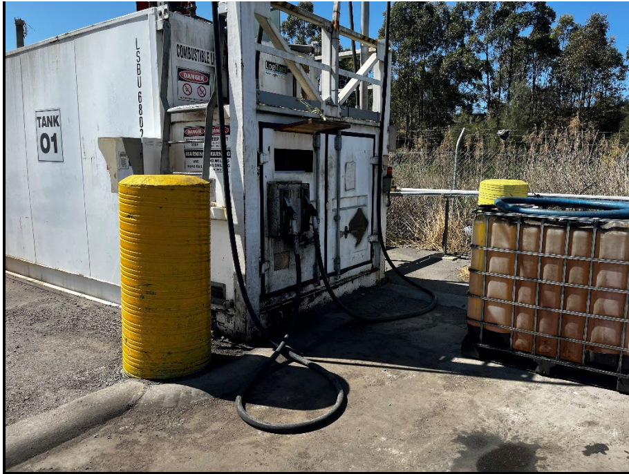
Photo 7: Self-bunded Diesel AST located in the southern corner of the site. Looking to the east.
