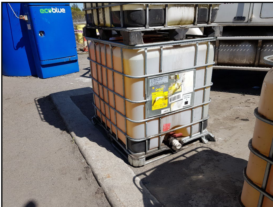
Photo 10: IBC reused to contain Diesel that is not labelled correctly located in the bund for the refuelling area.
