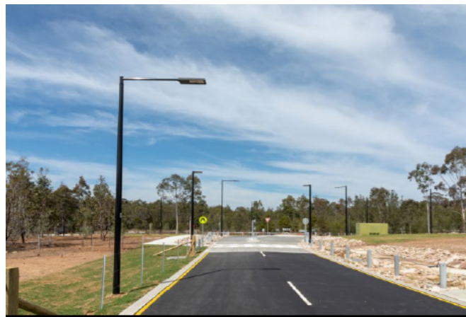
Street Lighting Pole (Source: WSPT Design Manual)
