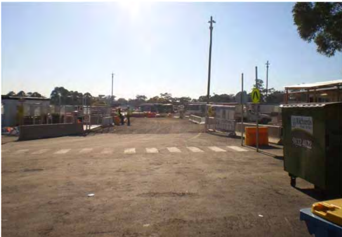
Photo 2 (August 2011) - Facing north-east with site office sheds to right of image
