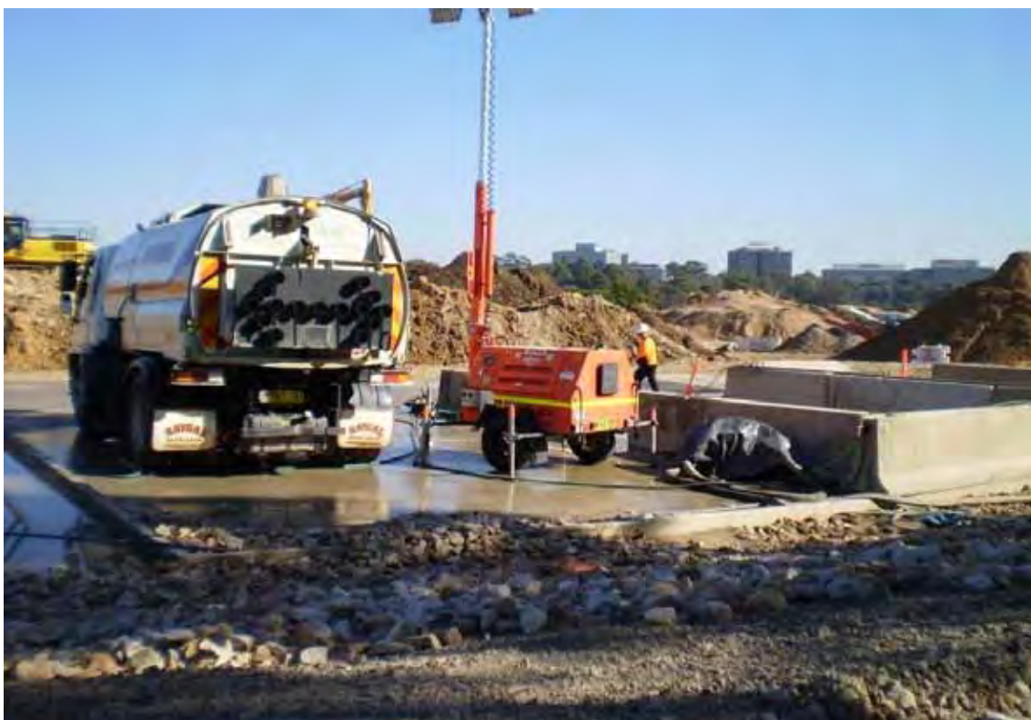
Photo 10 (August 2011) - Vehicle washbay facing north-west
