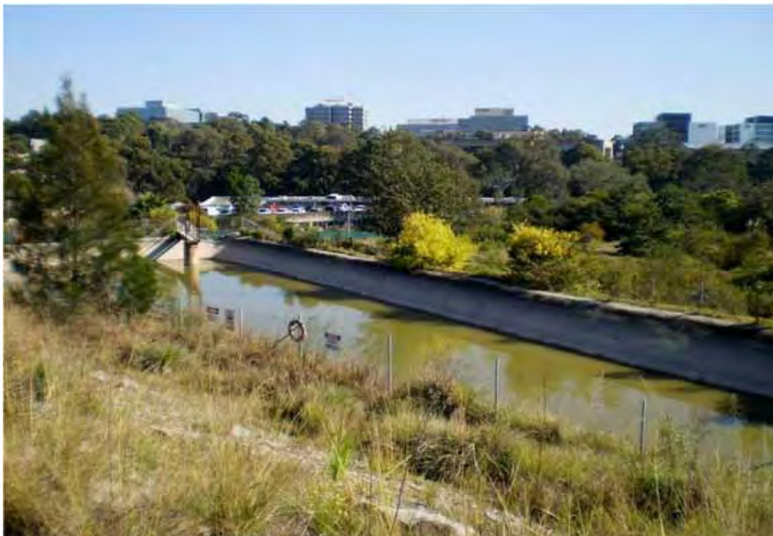
Photo 14 (August 2011) - Detention basin between compound stockpile area and bushland area
