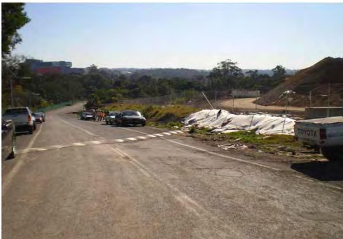
Photo 15 (August 2011) - North along site access road to the west of the compound
