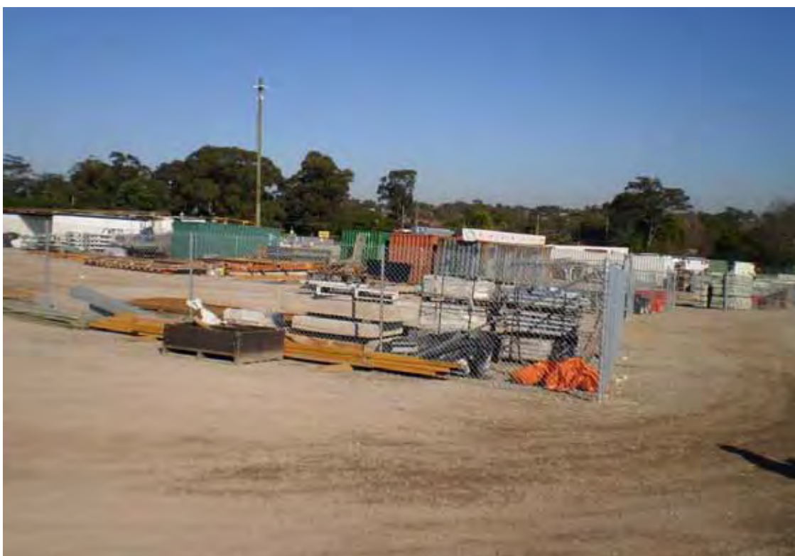
Photo 6 (August 2011) - Storage area within central area of Leighton compound
