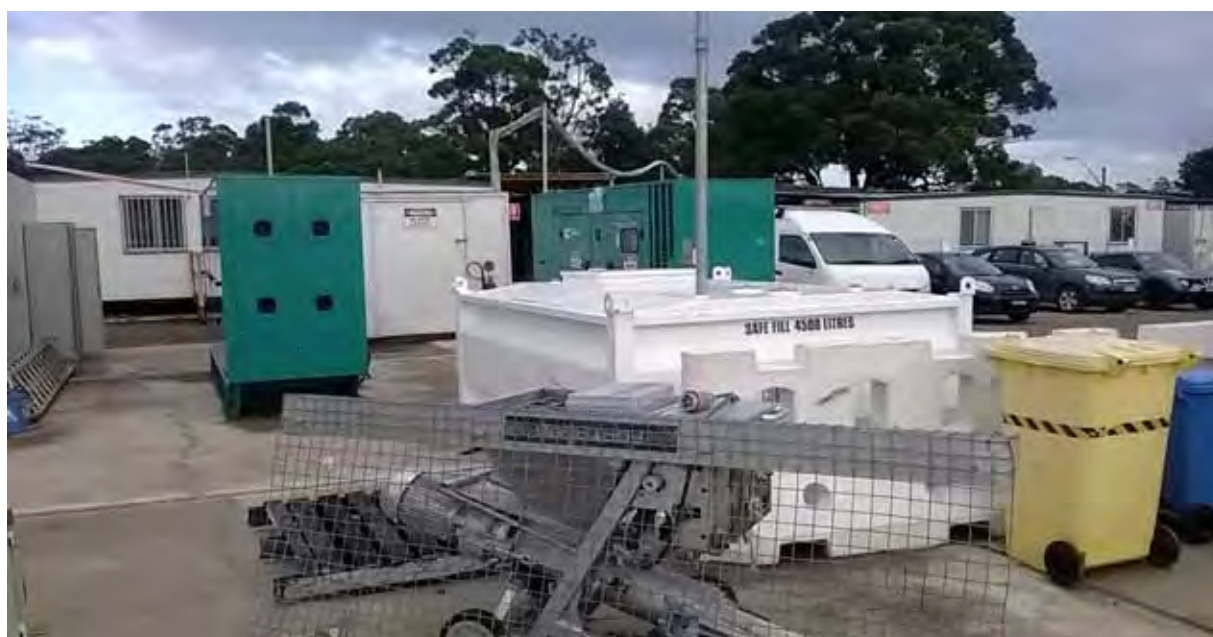
Photo 21 (15 April 2014) - Leighton generators and refuelling diesel tank on concrete slab
