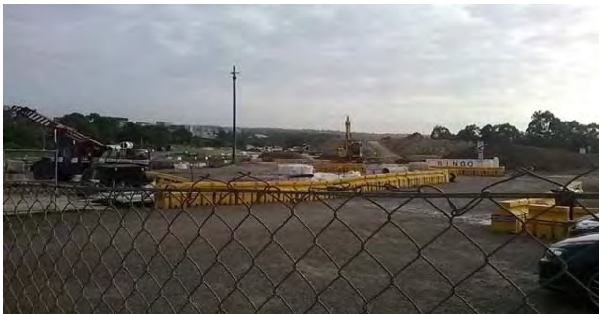
Photo 20 (15 April 2014) - view of Leighton and ETTT compounds
