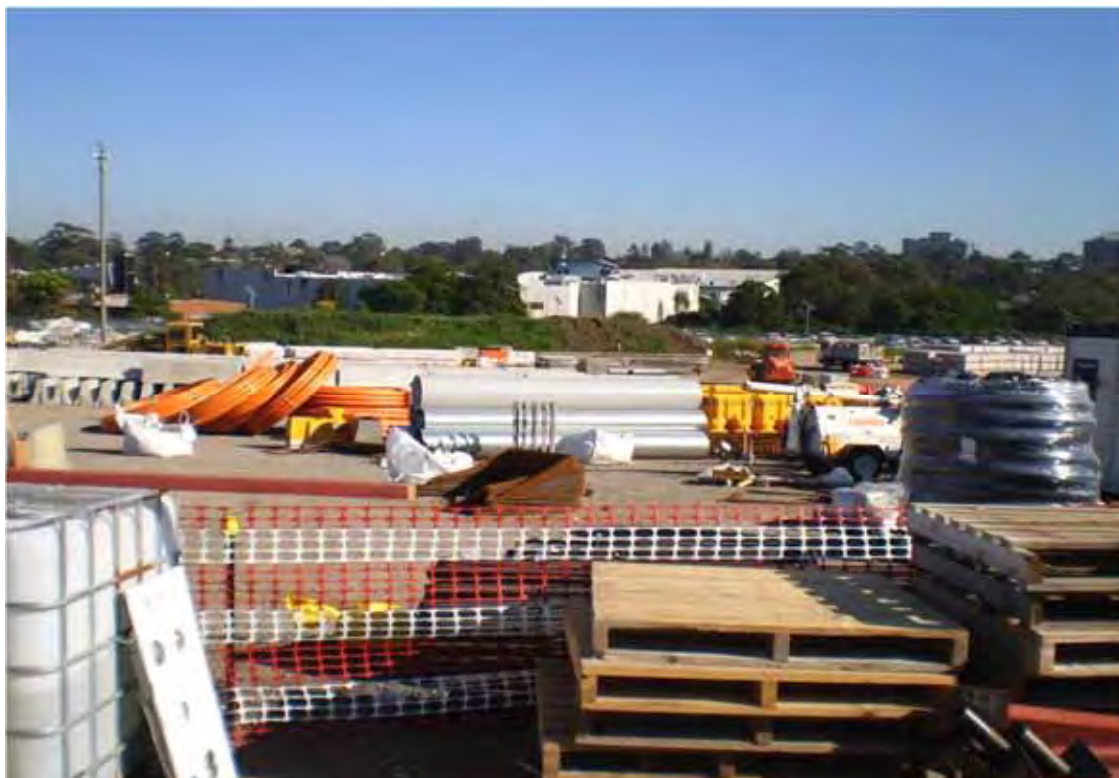
Photo 5 (August 2011) - Central area of Leighton storage compound
