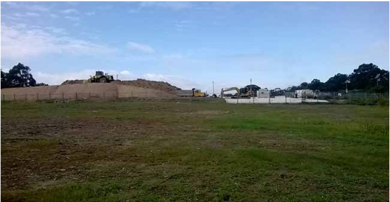
Photo 22 (15 April 2014) - cleared northern end of former Leighton compound
