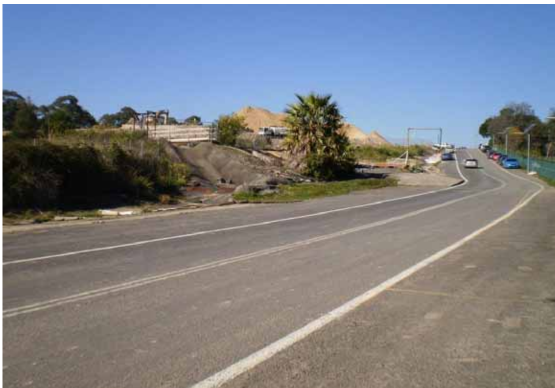
Photo 16 (August 2011)- South along site access road
