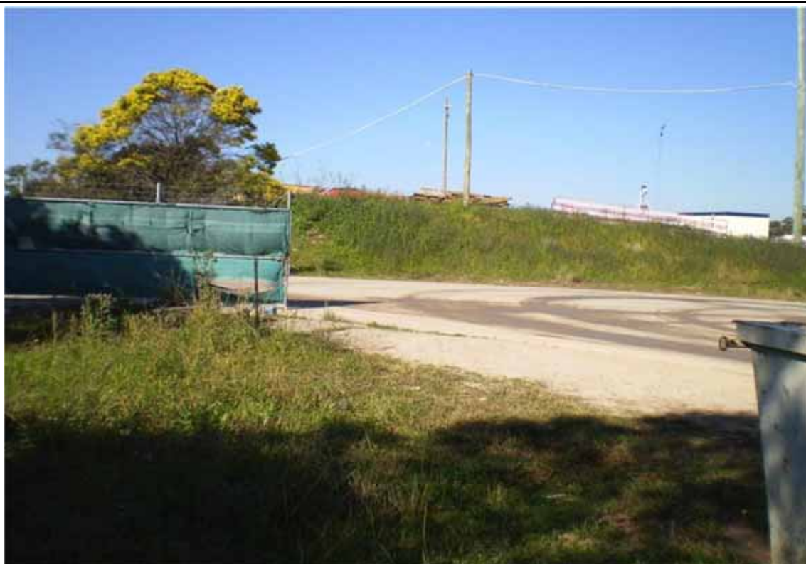
Photo 9 (August 2011) - Embankment at M2 access driveway facing south
