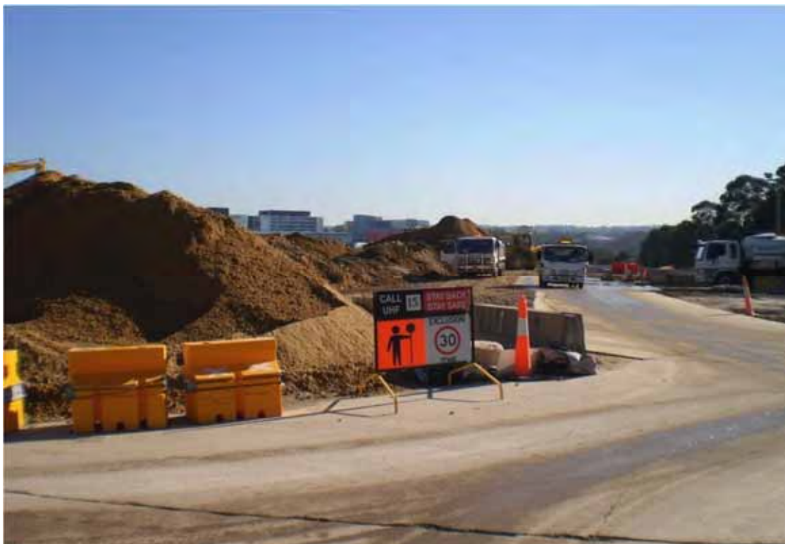
Photo 8 (August 2011) - Vehicle path along eastern side of stockpiles
