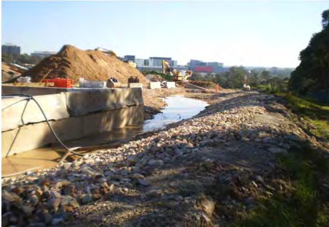
Photo 11 (August 2011) - Drainage of wash bay water towards north of stockpiles
