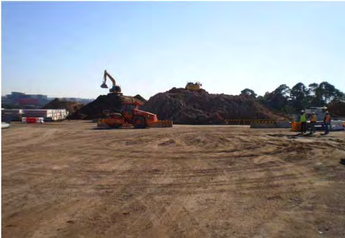
Photo 7 (August 2011) - Stockpiles generated from M2 Upgrade works
