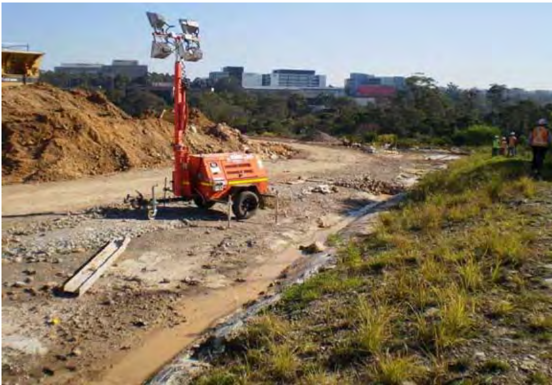
Photo 12 (August 2011) - Drainage of wash bay water towards sediment basin to the north
