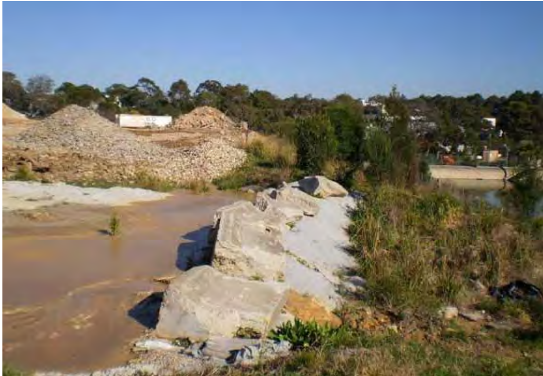
Photo 13 (August 2011) - Bunded sediment basin with large detention basin adjacent
