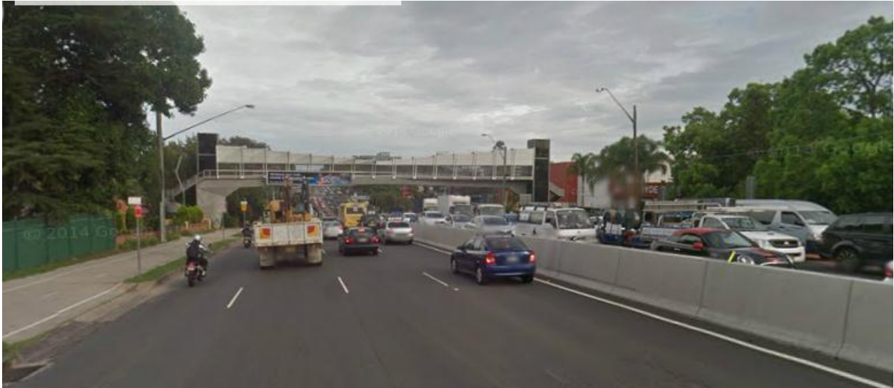
FIGURE 9 – VIEW NORTH ALONG EPPING ROAD TO PEDESTRIAN BRIDGE (SUBJECT SITE TO THE RIGHT)
