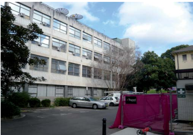
Figure 3.4 Area at the rear of the Physics Building (A28) where the proposed AIN Building is to be located. Demolition of the Physics Annex (A29), seen on the left, has been approved as part of a separate application
