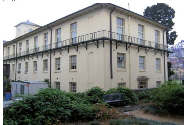
Figure 7.8 V28, view to the east face of the Physics Building
