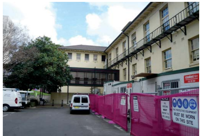
Figure 3.5 Partial view of the rear of the Physics Building (A28) where the proposed AIN Building is to be located
