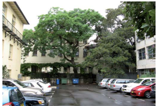
Figure 7.6 V21, view to the west elevation of the Edward Ford Building from the Physics carpark, prior to the loss of the jacaranda tree and pergola
