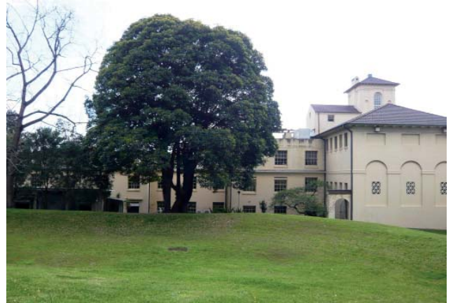
Figure 3.3 Partial view of the rear of the Physics Building (A28) where the proposed AIN Building is to be located
