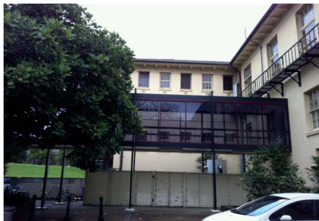
Figure 7.10 Photograph showing the building facades in the vicinity of the proposed eastern link where works are to be undertaken to comply with the fire separation requirements. The existing link to the Physics Annex has been approved for demolition as part of a separate application, with the exception of the remnant interface to the Physics Building
