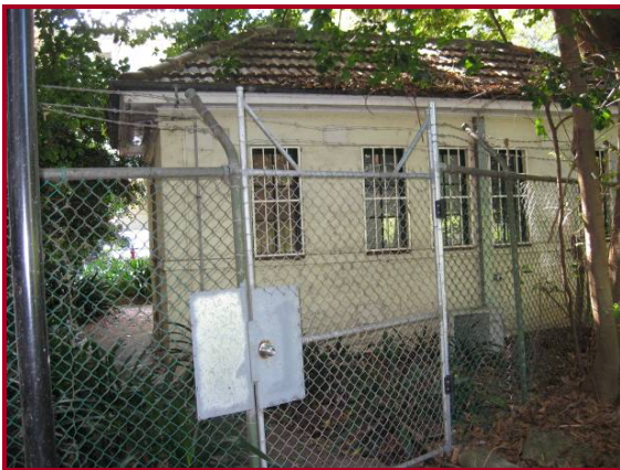
Figure 15. Flammable Store (A27C), looking east.
