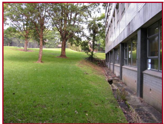
Figure 12. The southern wall of the Physics Annexe (A29).
