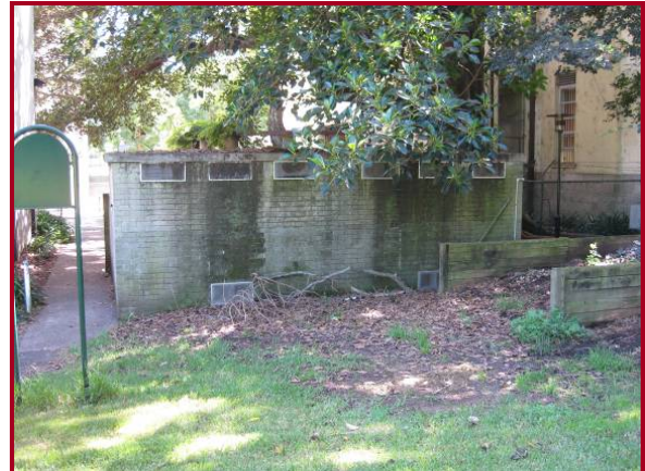
Figure 14. Flammable Store (A29A), looking north.
