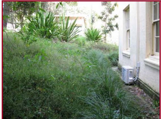
Figure 10. The southern wall of the Physics Building (A28).
