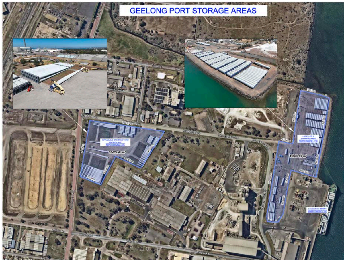
Figure 1 – Geelong Port Lascelles 3 and storage areas
