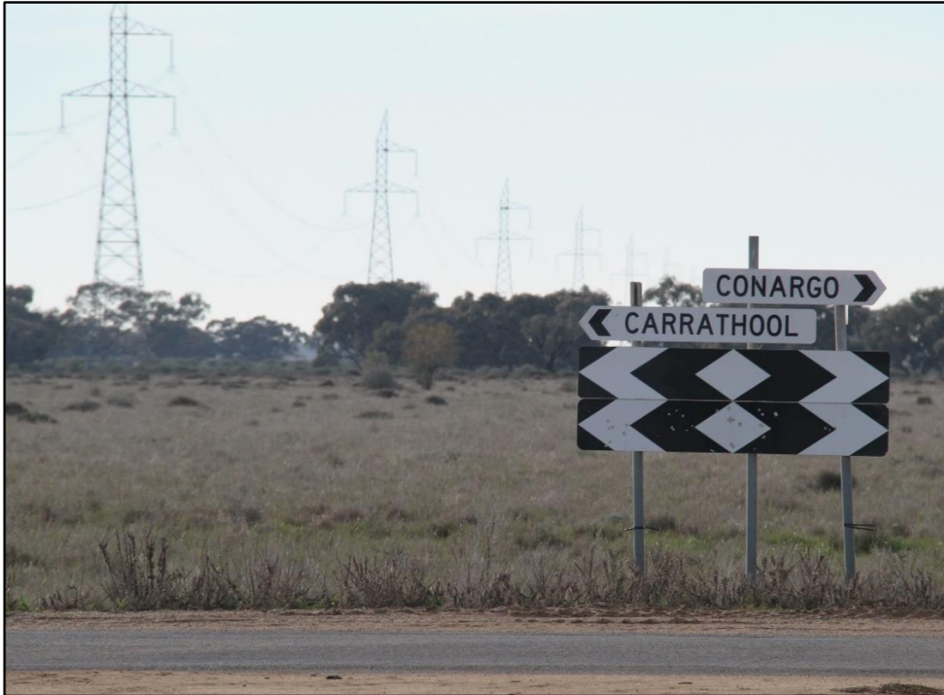
Figure 6 High Tension power line
