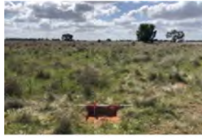
awan Wind Test Excavation (
