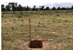
awan Wind Test Excavation (1
