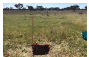
awan Wind Test Excavation (1
