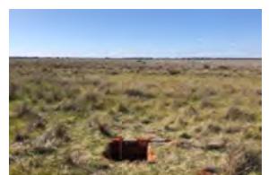
nawan Wind Test Excavation (3
