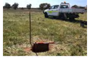
awan Wind Test Excavation (1
