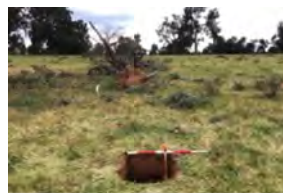
awan Wind Test Excavation (1
