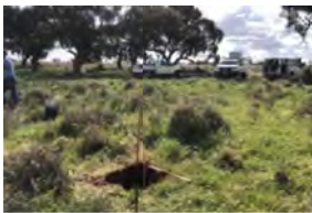
awan Wind Test Excavation (
