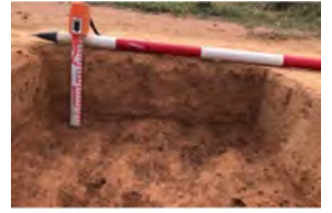
awan Wind Test Excavation (1)
