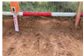
awan Wind Test Excavation (2
