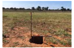
awan Wind Test Excavation (1
