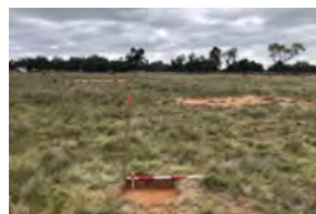
awan Wind Test Excavation (2)
