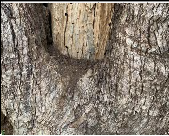
Description: Detailed close up of the bottom of the scar, revealing termite damage.
