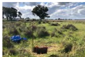
awan Wind Test Excavation (1
