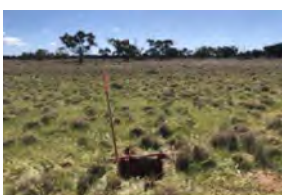
awan Wind Test Excavation (1
