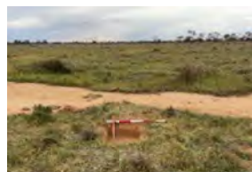
awan Wind Test Excavation (3
