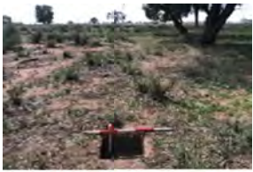
awan Wind Test Excavation (
