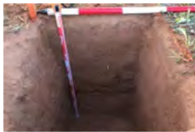
awan Wind Test Excavation (1
