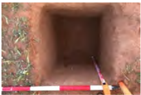
awan Wind Test Excavation (1
