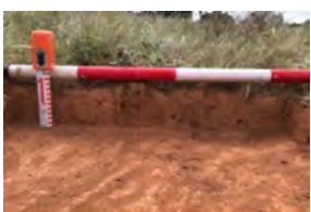
awan Wind Test Excavation (2)
