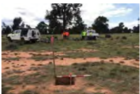
awan Wind Test Excavation (1
