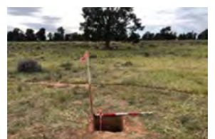
awan Wind Test Excavation (1
