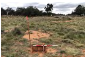
awan Wind Test Excavation (2)
