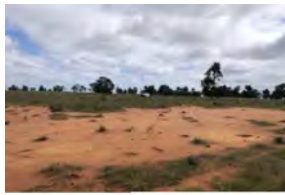
awan Wind Test Excavation (1)
