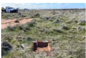
awan Wind Test Excavation (2
