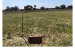
awan Wind Test Excavation (1
