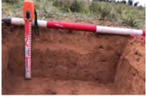
awan Wind Test Excavation (1)
