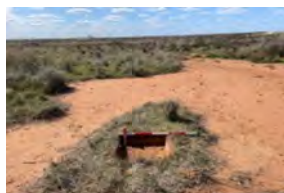
awan Wind Test Excavation (2
