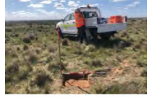
awan Wind Test Excavation (2
