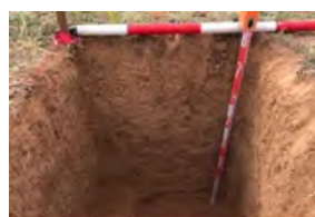
awan Wind Test Excavation (1
