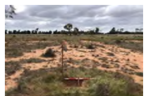
awan Wind Test Excavation (2)
