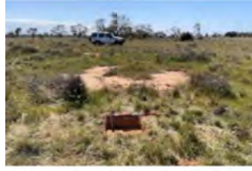
awan Wind Test Excavation (2
