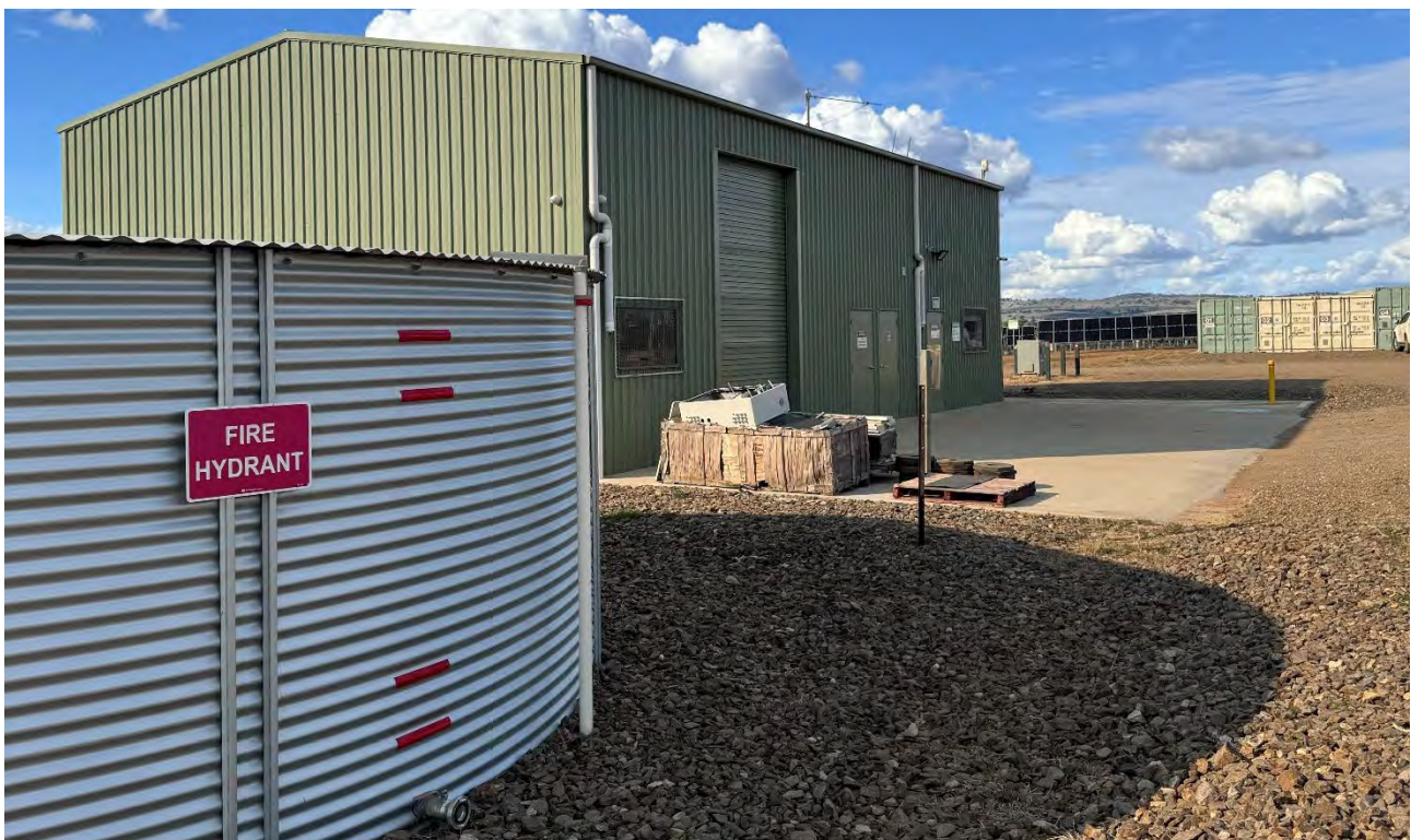
Photograph 3.3 Example of an operations and maintenance facility
