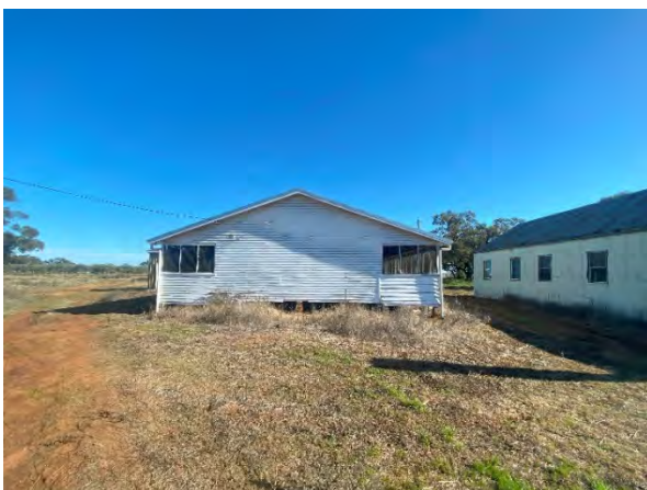
Plate A.30 Building C of DEHW002, a weatherboard structure elevated by brick piers. View west.
