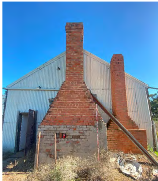
Plate A.25 Two brick fireplaces located outside the kitchen area of Building A, connecting to wood stove and fireplace in kitchen. View west.
