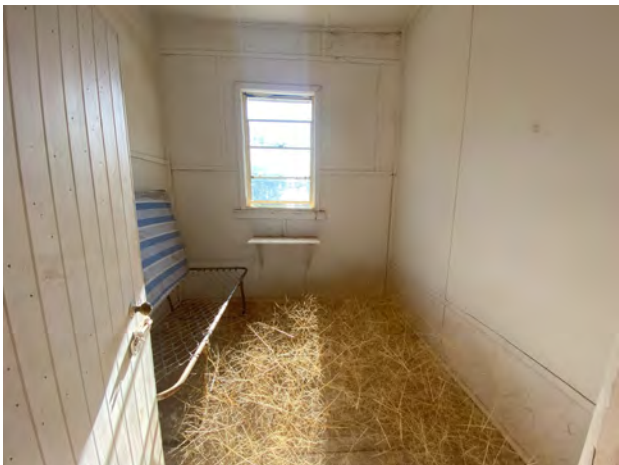
Plate A.20 Bedroom interior in Building A showcasing timber floorboards, a window, and a bedframe with a mattress. Similar rooms are found throughout the building. Blown grass visible on the floor. View south.
