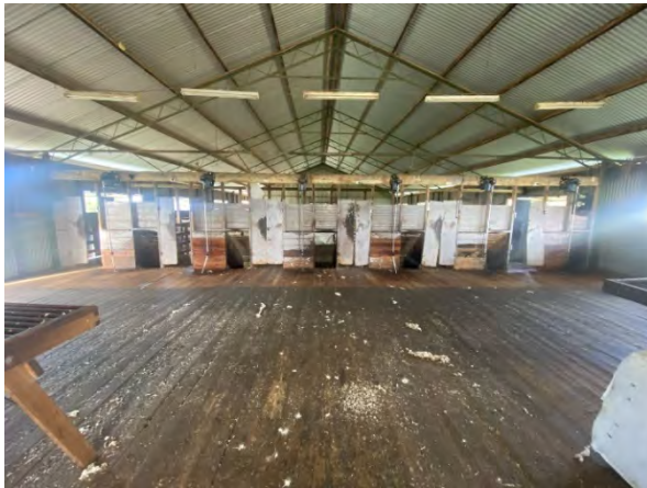
Plate A.44 Internal view of woolshed, internal renovations include new flooring. View south.
