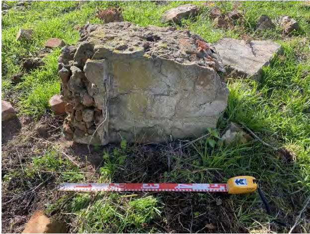
Plate A.52 Detail of a collapsed rendered brick ruin with an in situ concrete foundation in the background. Interpreted as possible chimney remains. View east.
