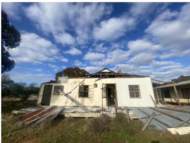
Plate A.42 Original weatherboard dwelling within DEHW004 now abandoned and in a state of disrepair. View south.
