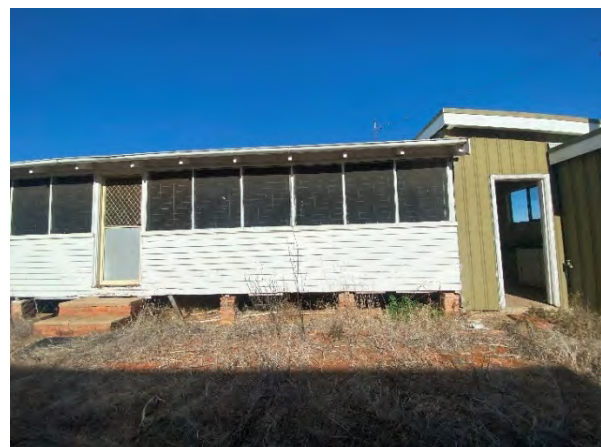
Plate A.31 Detail of Building C showing steps leading to the main entrance, along with the green vinyl extension housing the laundry and bathroom area. View south.
