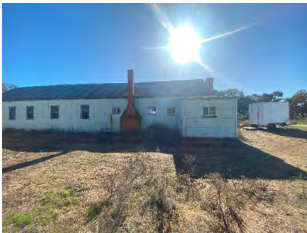
Plate A.16 Building A of DEHW002, showing a brick fireplace and corrugated iron clad exteriors. This building accommodates the kitchen, dining area, and bedrooms, with the pantry visible in the foreground as a return in the structure. A portable refrigeration unit is positioned to the east. View north.
