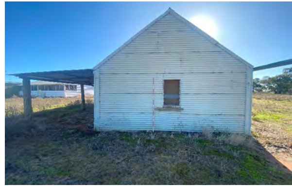
Plate A.27 Building B of DEHW002. The single window is covered, obstructing views inside. View north.
