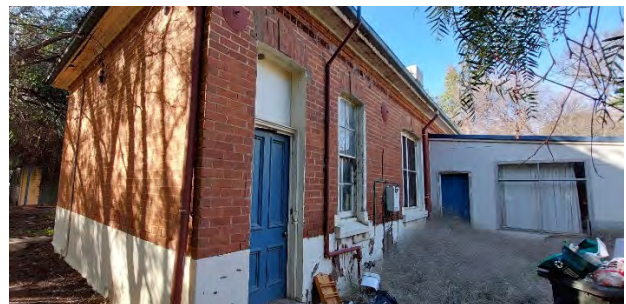
Plate A.2 Dry pressed brick dwelling with plasterboard extension within the Goolgumbla complex (DEHW001), view north-west.
