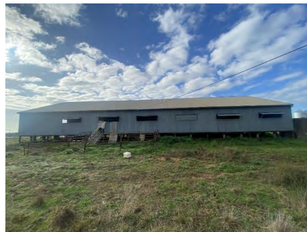
Plate A.43 Woolshed situated within DEHW004, highlighting external renovations that have been undertaken, including the installation of a new roof. View east.
