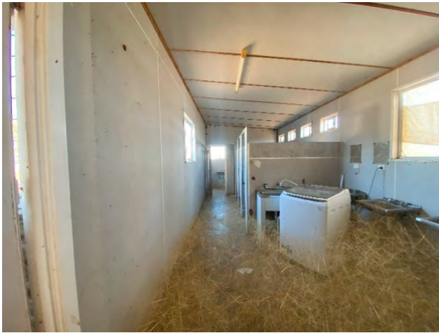
Plate A.32 Interior of the extension of Building C, revealing metal basins, a washing machine, and shower and toilet cubicles. Blown grass covers the floor of this area. View south.
