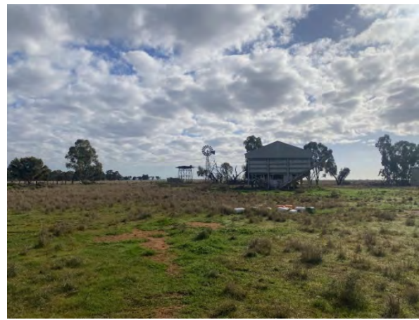
Plate A.47 East-facing view of DEHW004 with water tank, tank stand and windmill.
