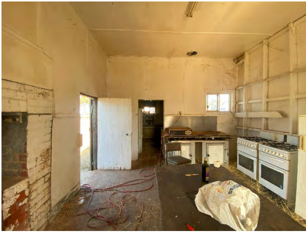
Plate A.18 Kitchen interior of Building A, showing a brick fireplace with wood stove insert to the east, alongside modern kitchen amenities to the west. A doorway leading to the pantry is visible in the background. View south.
