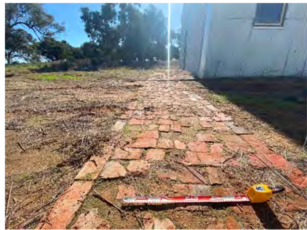
Plate A.17 Example of sandstock brick paving arranged in a running bond pattern. Located on the western end of Building A. View north.
