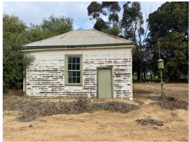
Plate A.8 Detail of weatherboard outbuilding within the Goolgumbla complex (DEHW001), view south.
