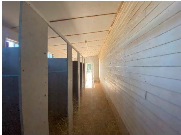
Plate A.33 Detail of toilet and shower cubicles within Building C. View north.
