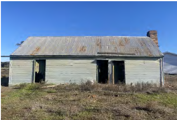
Plate A.28 Three small back rooms in Building B of DEHW002, featuring broken timber doors. These compact spaces may have served as storage areas. View west.
