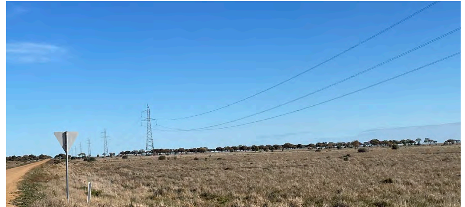
Image 30 – Existing 220 kV transmission towers within Study Area
