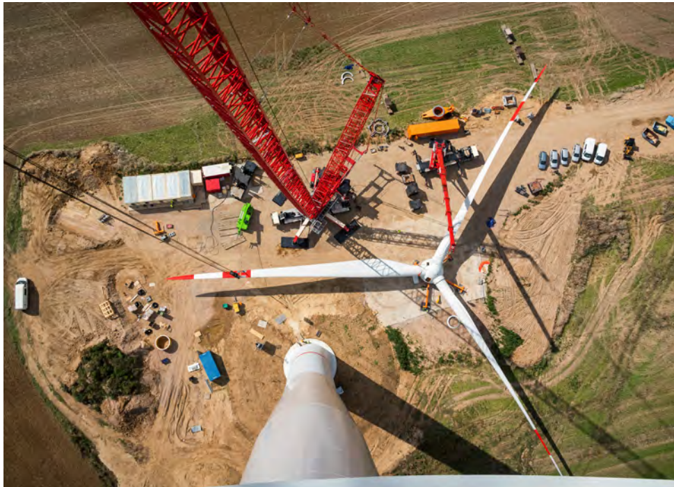
Image 03 – Crane Hardstand (Source: EMM)
