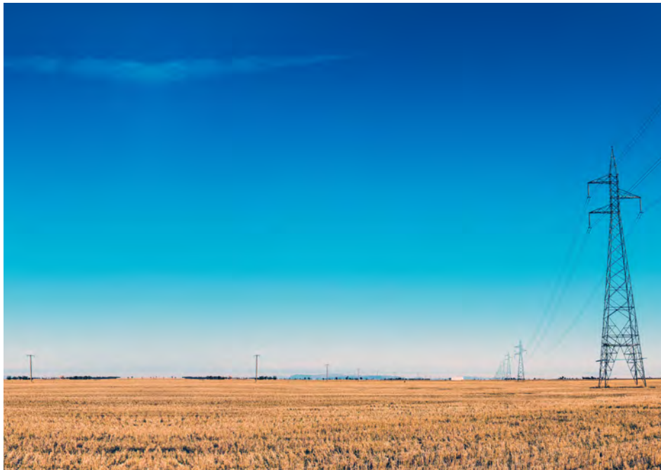
Image 04 – Transmission Line (Source: EMM)
