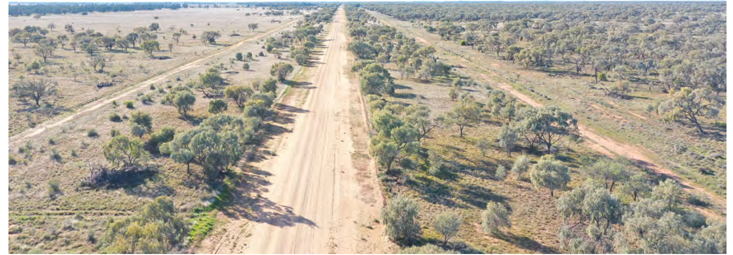
Image 14 – View over McLennons Bore Road Image Source: Moir LA , 2023
