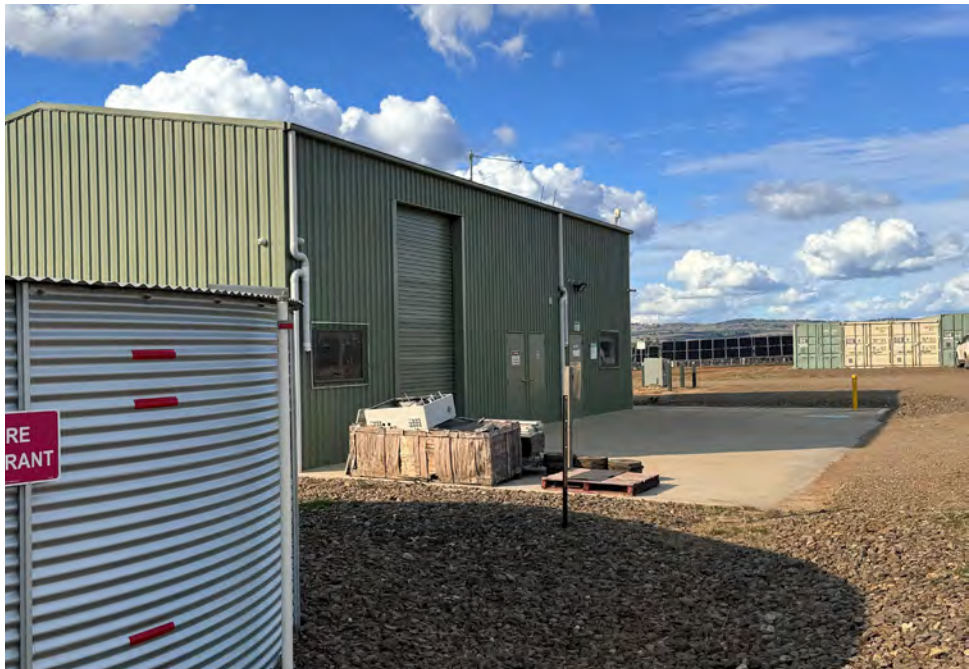
Image 05 – Operations of Maintenance Facility (Source:Spark Renewables)
