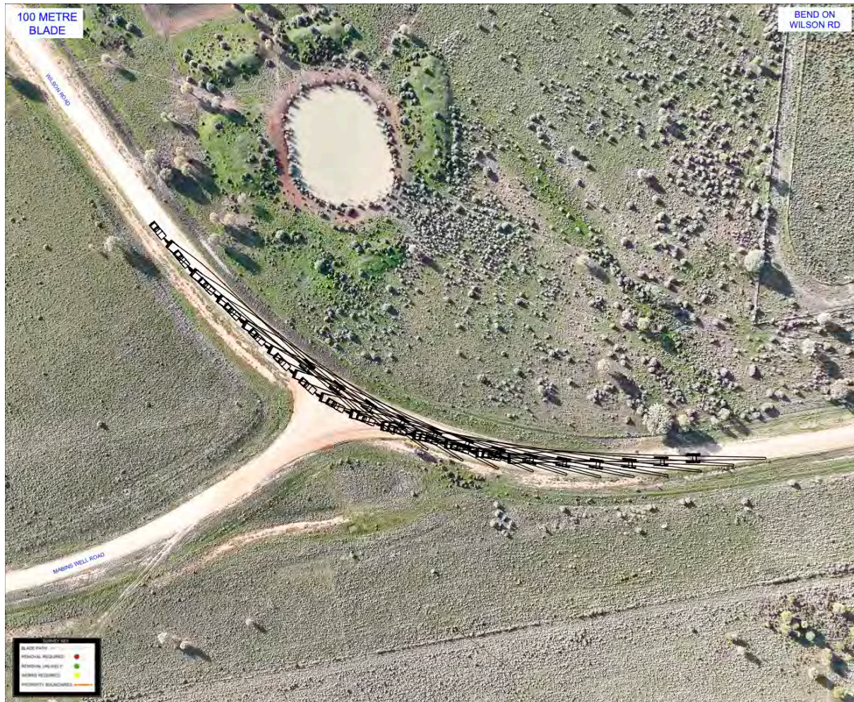
Figure 34 - Bend on Wilsons Rd
