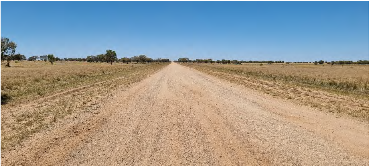
Plate 3.3 McLennons Bore Road
