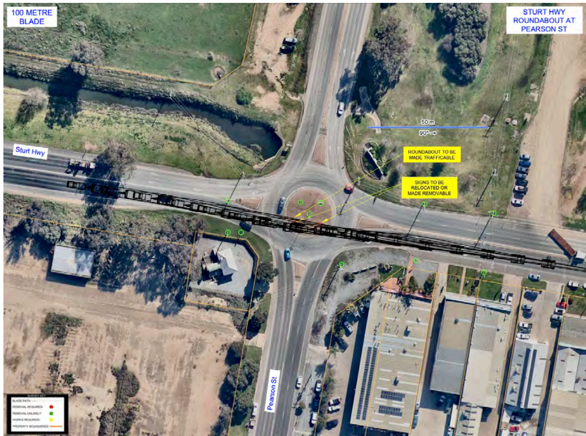
Figure 29 - Sturt Hwy Roundabout at Pearson St
